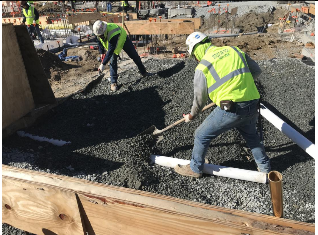
Photo 4: View of STNY placing the permeable aggregate layer for the SMD system in waste characterization grid COMP A (facing north)
