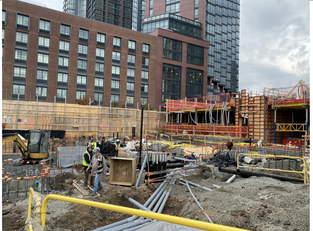
Photo 1: General view of the site (facing west).
