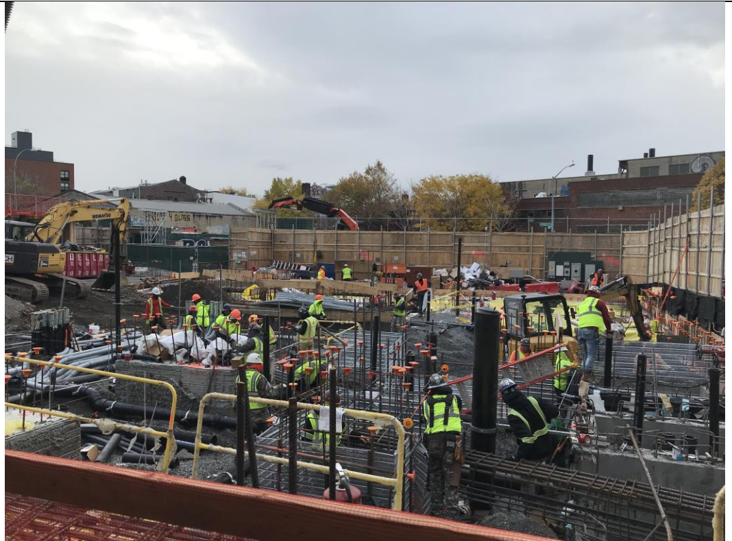
Photo 1: General view of the site (facing south).
