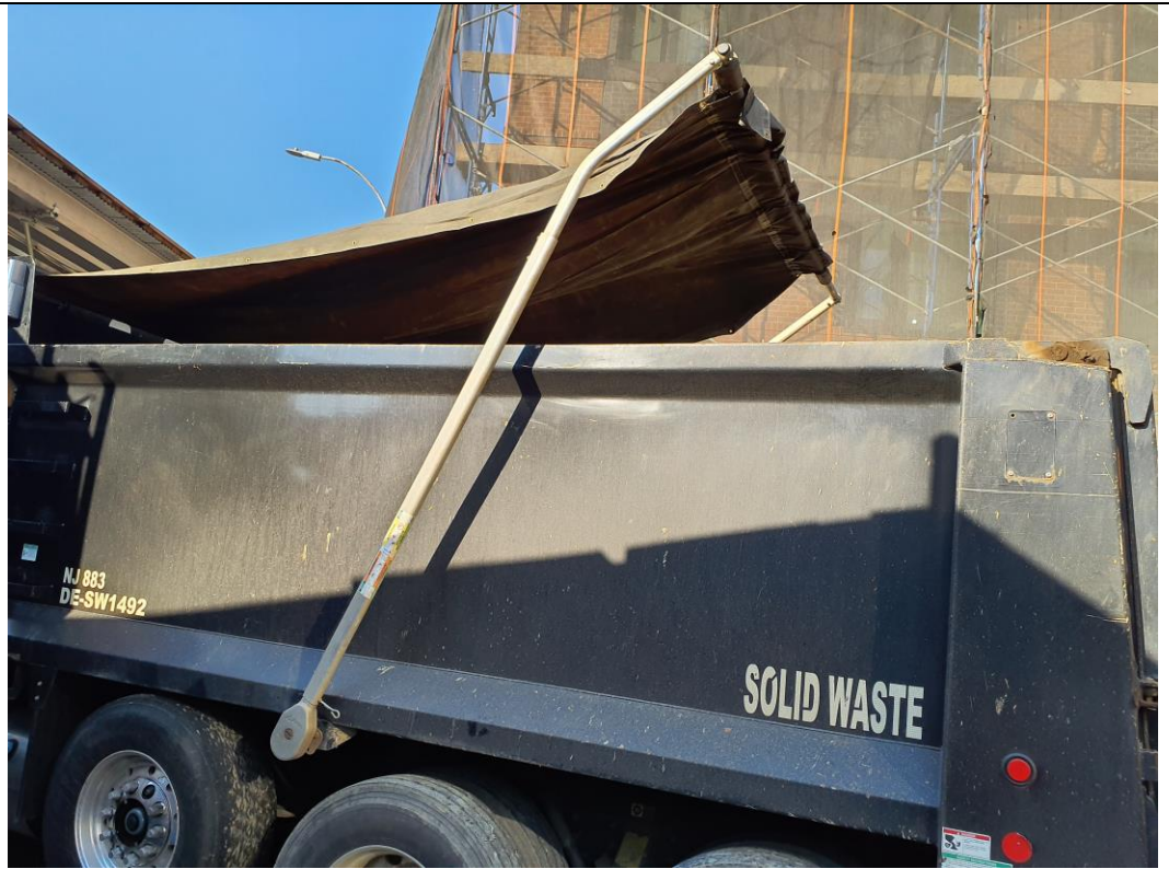
Photo 4: View of loaded truck being secured prior to leaving the site (facing southwest).
