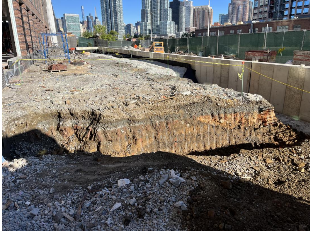
Photo 3: View of the retaining wall excavation (facing north).
