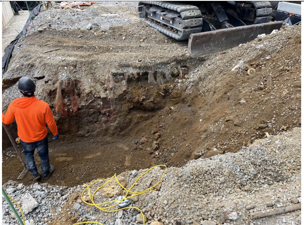
Photo 4: View of the retaining wall excavation (facing south).
