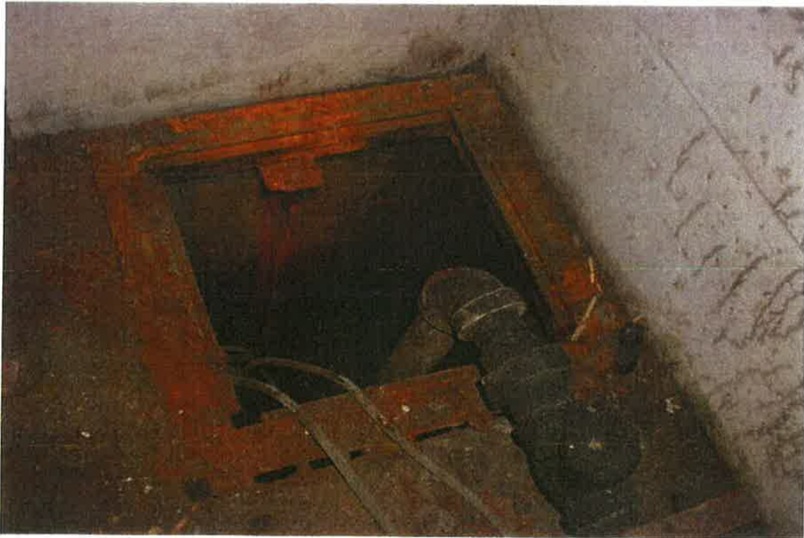
3. View of a typical storm water catch basin during the dye testing activities.
