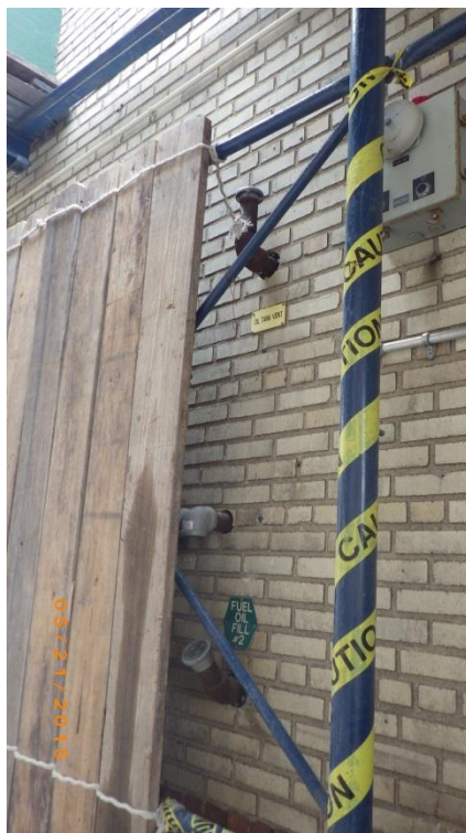
Photograph 14: View of vent pipe and fill port at northern face of southwestern adjoining building.
