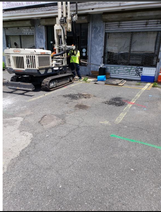
Installing Soil Boring SB-3
