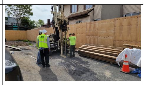
Photo 4 –Depicts the installation of a 2-inch groundwater monitoring well.
