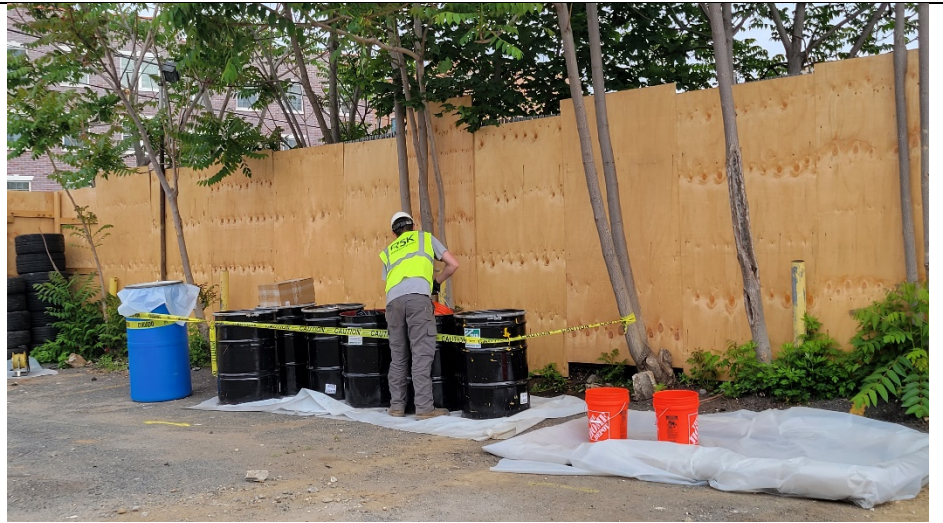
Photo 3 –Depicts purged groundwater being containerized on-site into DOT-approved 55-gallon drums.
