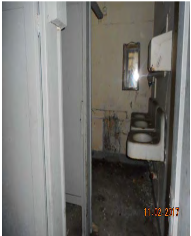
Second floor- bathroom
