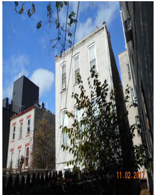
Adjacent residential buildings to the north
