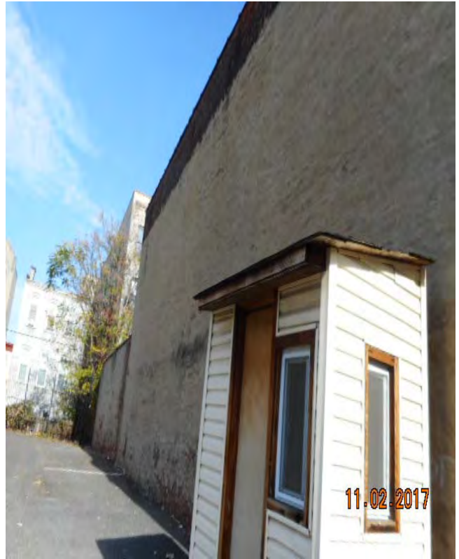
Parking lot- Security post
