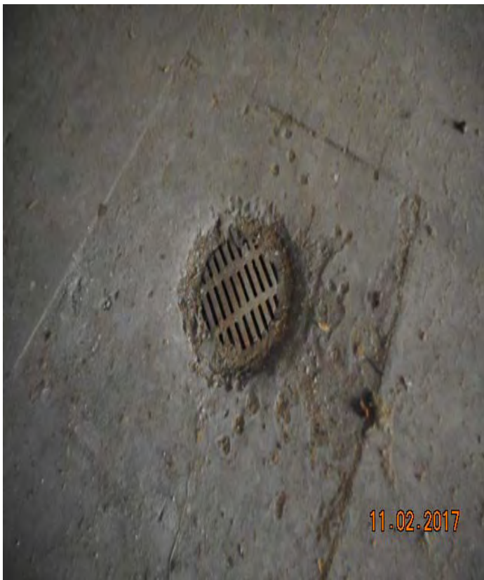
Second floor-floor drain
