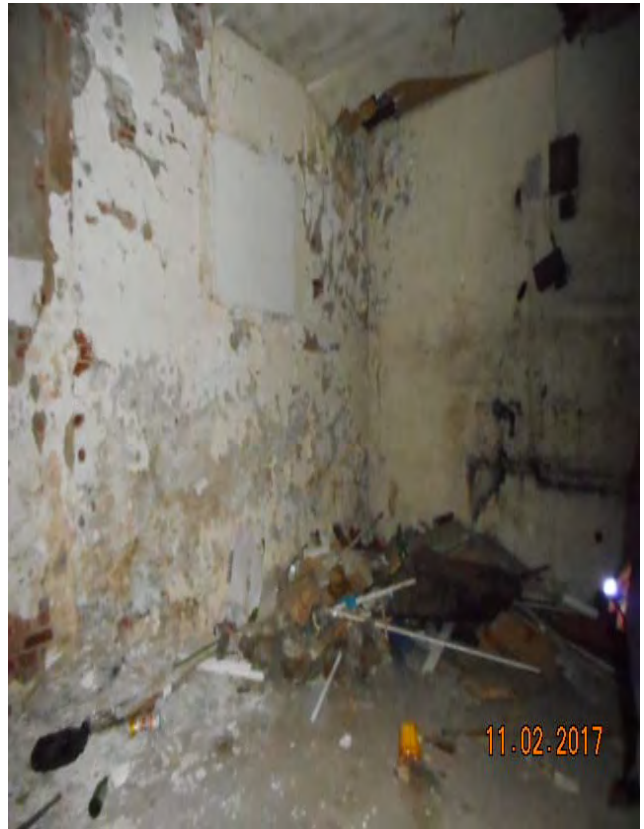
First floor- northern portion of the subject building
