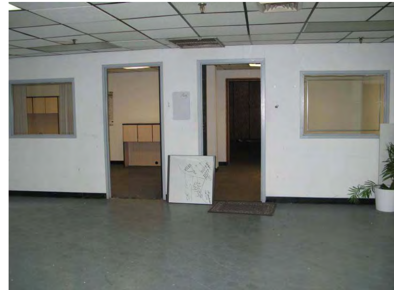
Photo 20: Office area at east end of 473-491 President Street building.
