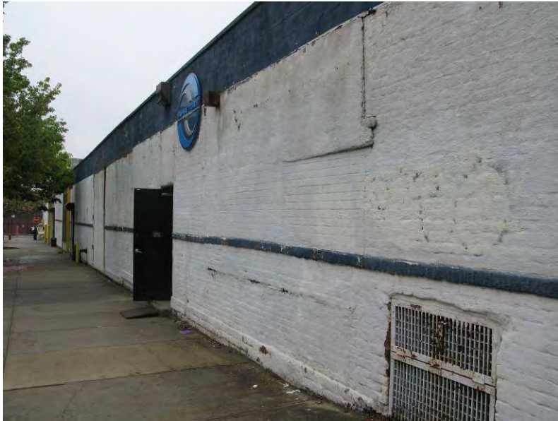
Photo 13: Looking northwest at the 473-491 President Street building.
