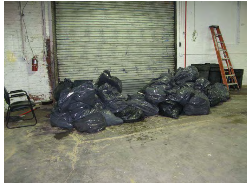
Photo 16: Trash storage inside the 473-491 President Street building.
