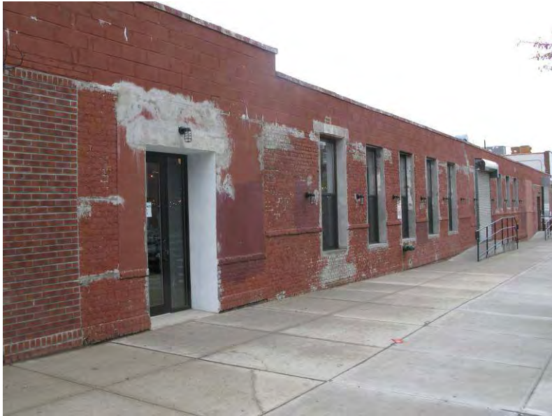
Photo 5: Looking southwest at the 514 Union Street property.
