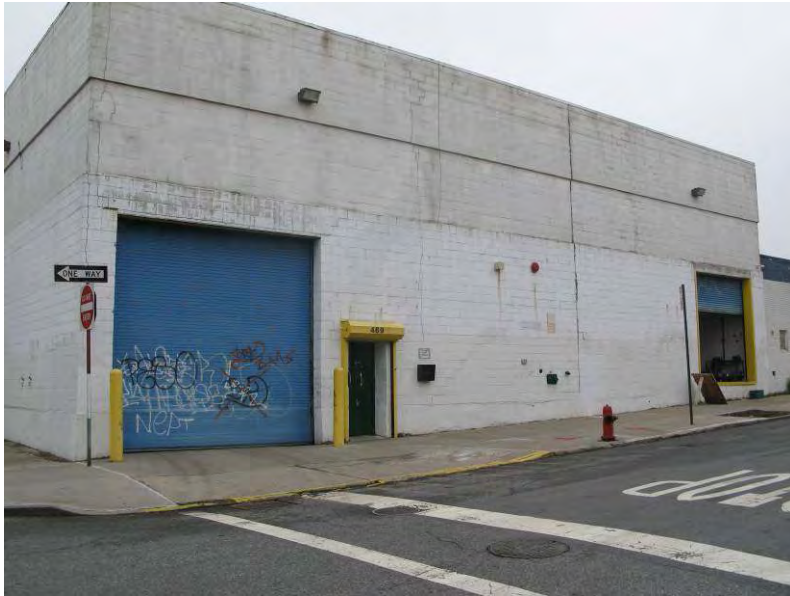
Photo 9: Looking north at the President Street/Nevins Street building.
