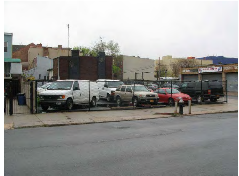
Photo 2: Looking southeast at the Nevins Street/Carroll Street lot.
