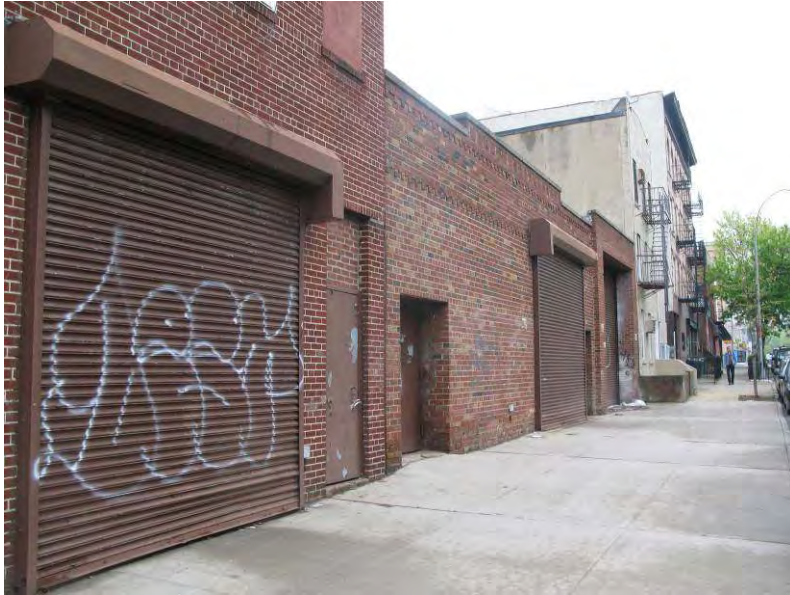
Photo 25: President Street to the east of the site.
