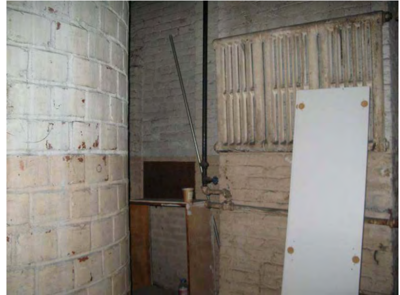
Photo 18: Mechanical room with remains of brick smokestack (left).
