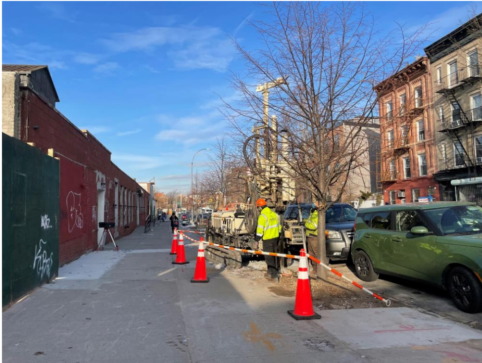
Photo 1: AARCO advancing soil boring EB17 on the Union Street sidewalk (facing west)
