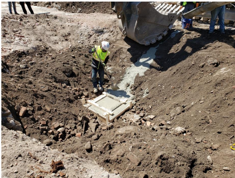
Photo 2: Kingdom placing concrete to install a foundation pile cap in the eastern part of the site (facing southwest)
