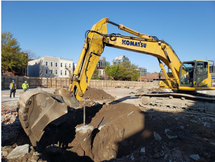
Photo 1: Kingdom excavating an area to install a foundation pile cap in the eastern part of the site (facing southwest)
