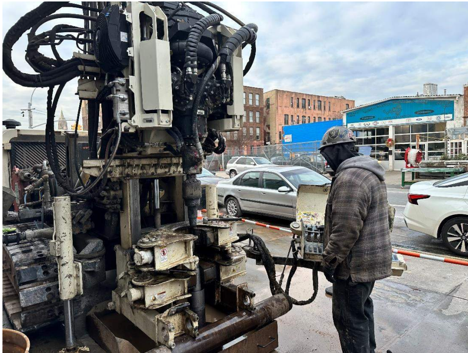
Photo 11: Eastern advancing sidewalk boring SB01_CT near MW-12S in the Union Street sidewalk (facing north) 12/27/2022
