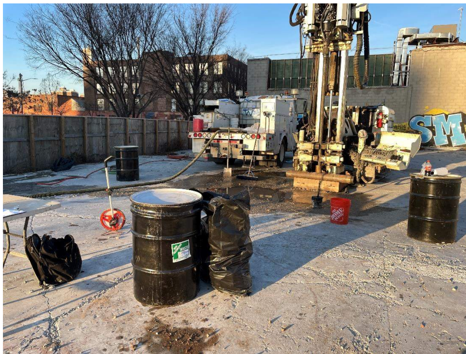
Photo 6: Drums of investigation-derived waste (IDW) staged near boring SB02_CT (facing north) 12/21/2022
