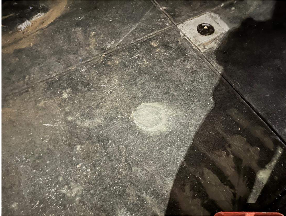
Photo 13: Sidewalk boring location SB01_CT repaired before demobilization 12/27/2022
