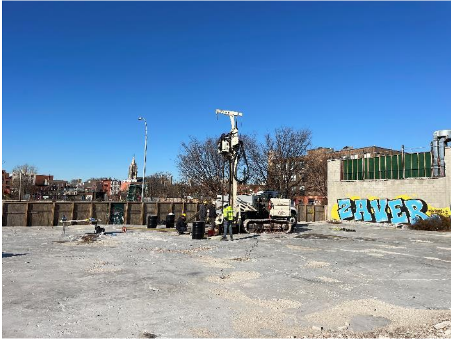
Photo 1: Eastern Environmental advancing soil boring SB02_CT in the western part of President Street Portfolio (facing north)
