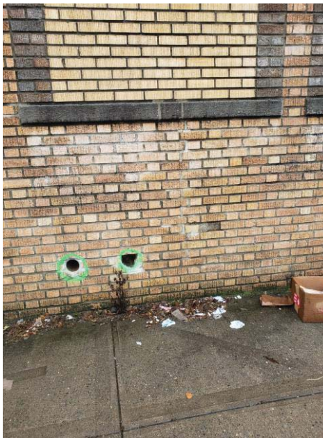
Photo #9 - Missing bricks and holes observed in the exterior perimeter wall at lot 26 & 28. Cause of possible water infiltration and structural deficiency in masonry wall.
