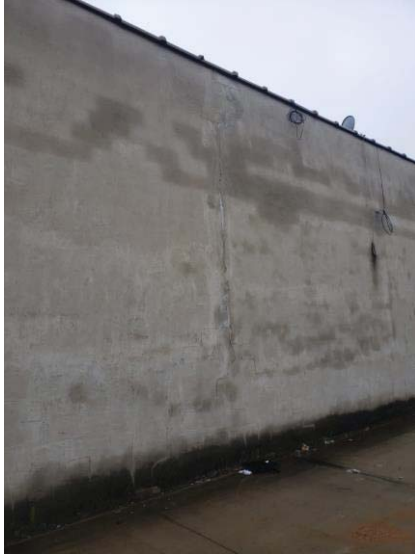
Photo #1 - Cracks in exterior wall along lot #17. It appears that settlement has occurred at the exterior wall.
