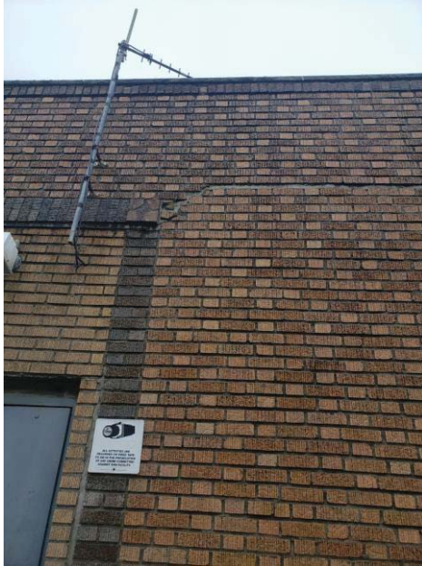
Photo #7 - Cracks above exterior door lintel at lot 26 in the exterior masonry wall. Cracks appear to be caused by settlement. The mortar in the masonry joints is also missing in areas.
