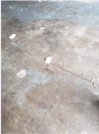
Photo #4 - Cracks observed in the slab on grade at lot 26 & 28. Slab appears to be in disrepair.
