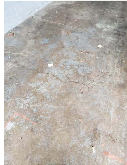
Photo #5 - Additional cracks observed in the slab on grade at lot 26 & 28. Slab appears to be in disrepair.
