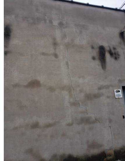
Photo #2 - Additional cracks in exterior wall along lot #17 at the parking lot. It appears that settlement has occurred at the exterior wall.
