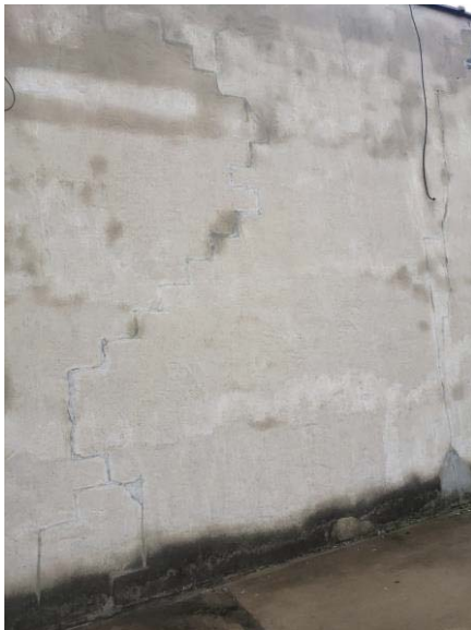
Photo #3 - Additional cracks in exterior wall along lot #17 at the parking lot. It appears that settlement has occurred at the exterior wall.
