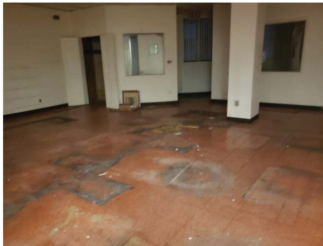
Photo #6 - Uneven and settling slab on grade observed in the slab on grade at lot 17. Slab appears to be in disrepair. The linoleum floor tile appears to be lifting and cracking which could be caused by the settling, or by moisture infiltration through the slab.
