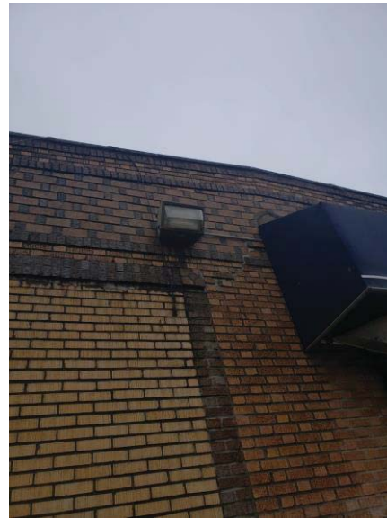
Photo #8 - Additional cracks observed above exterior door lintels at lot 26 & 28 in the exterior masonry wall. Cracks appear to be caused by settlement.
