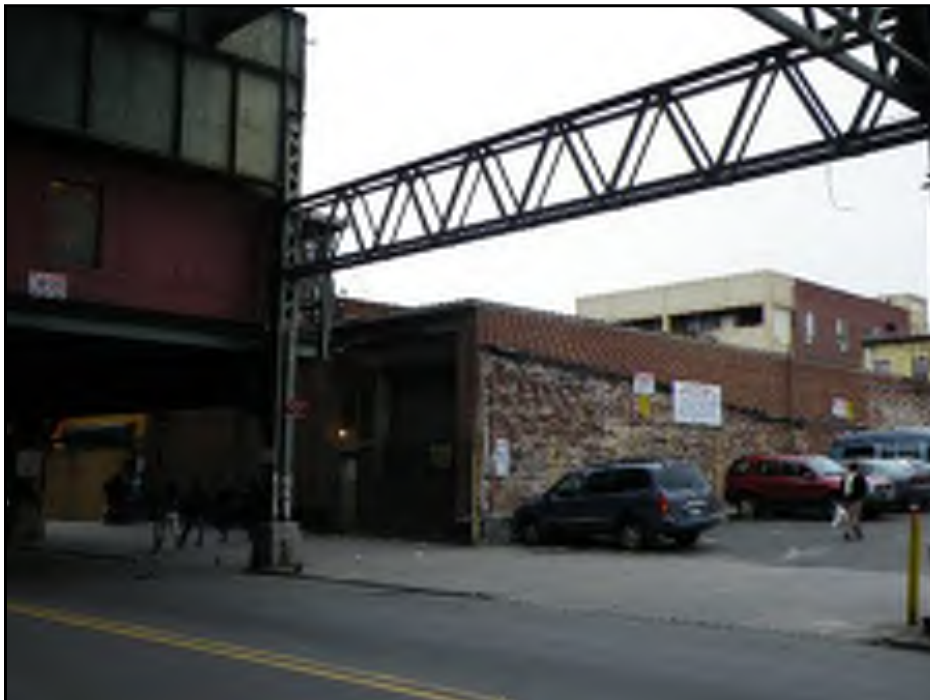
Eastern adjoining NY Transit Substation
