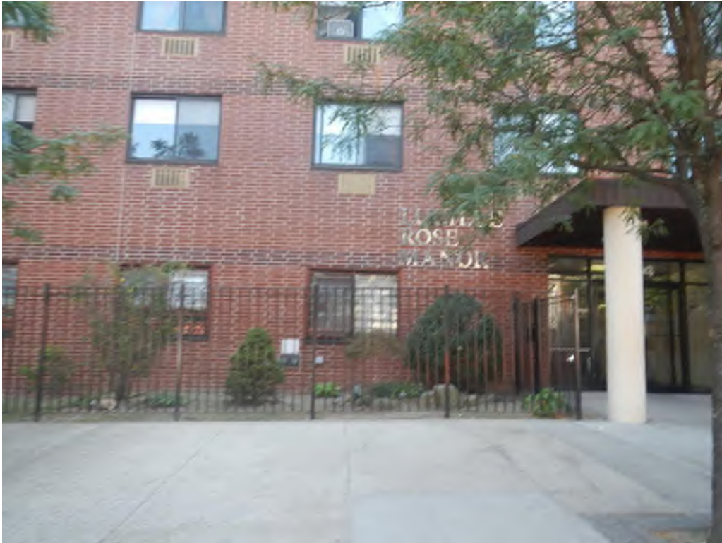
Residential apartment building to the south of Vernon Avenue
