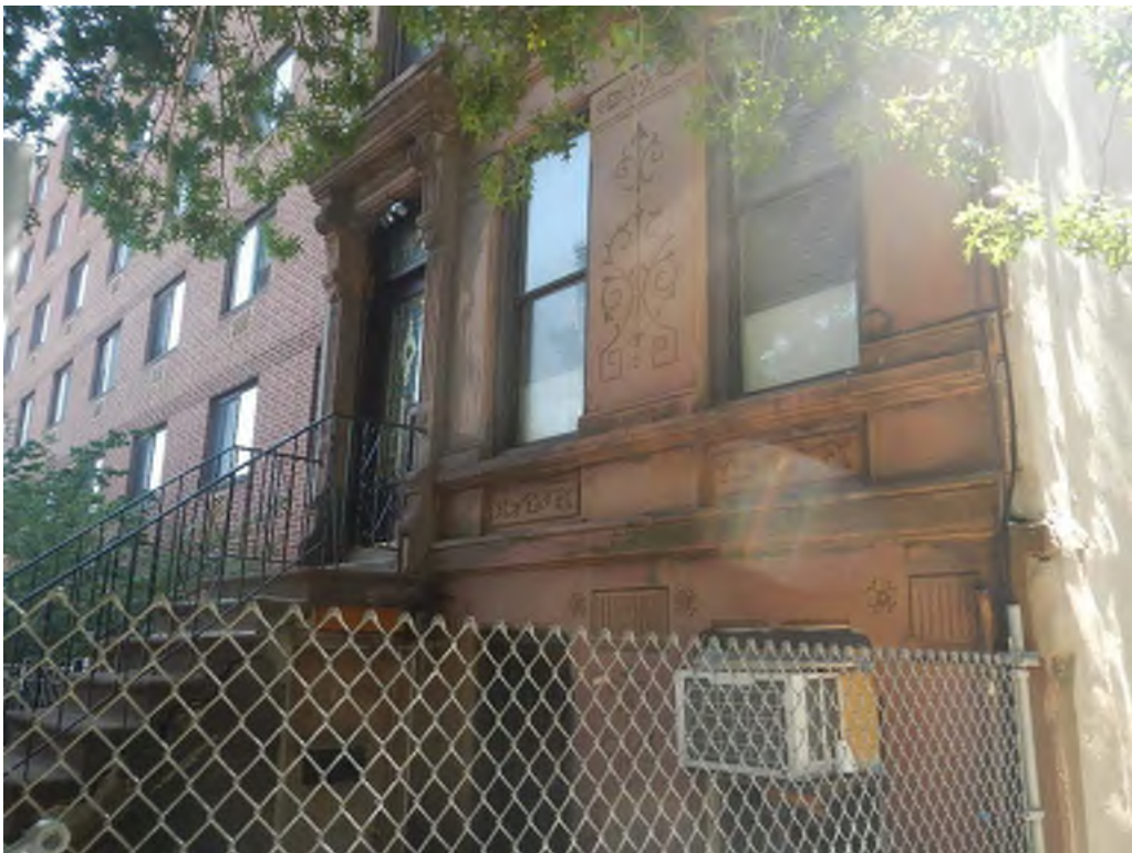
Adjoining residential properties observed along Vernon Avenue
