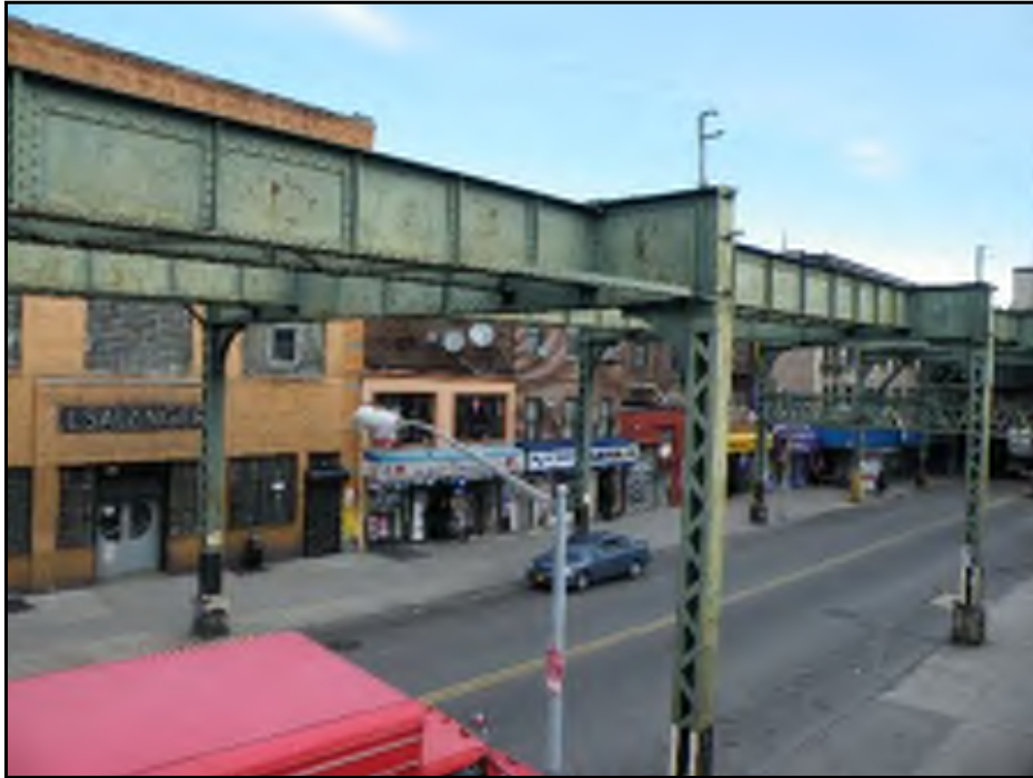
Northern adjoining commercial development
