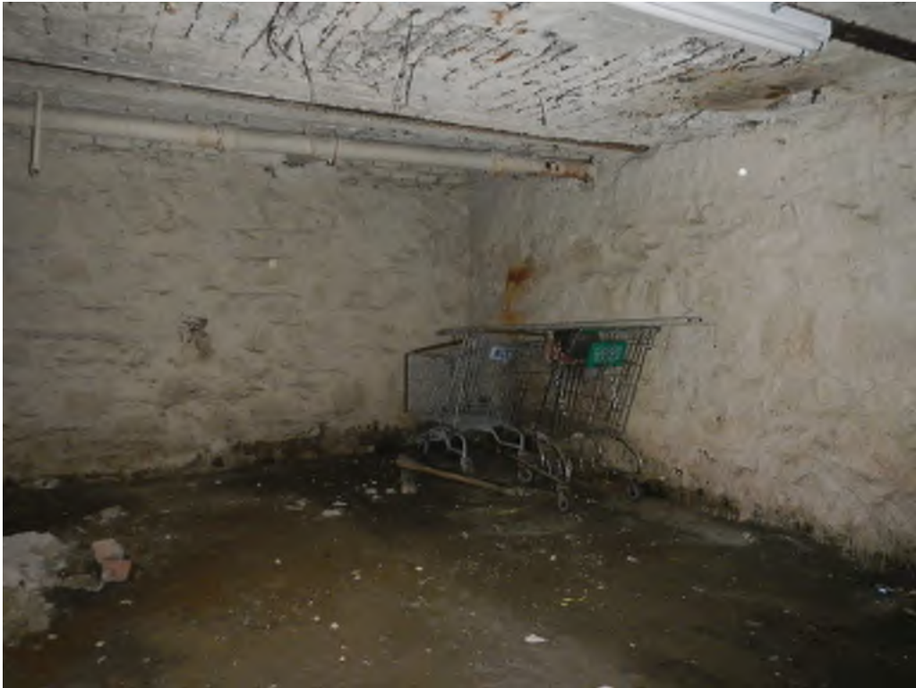
The partial basement area of the Property
