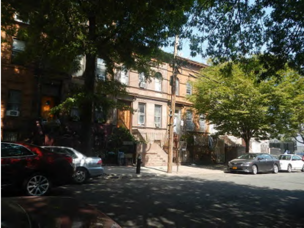
Residential properties observed along Vernon Avenue
