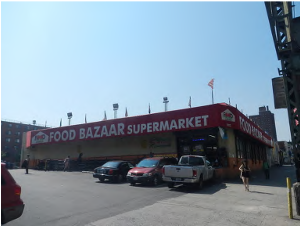
The Property viewed from the northeast along Myrtle Avenue
