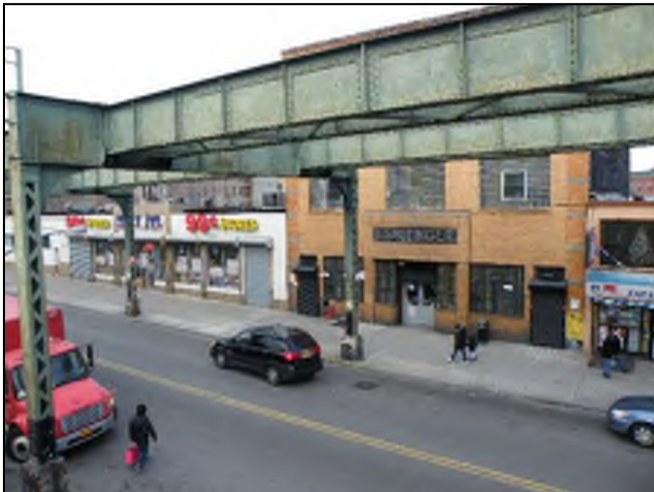
Northern adjoining commercial development
