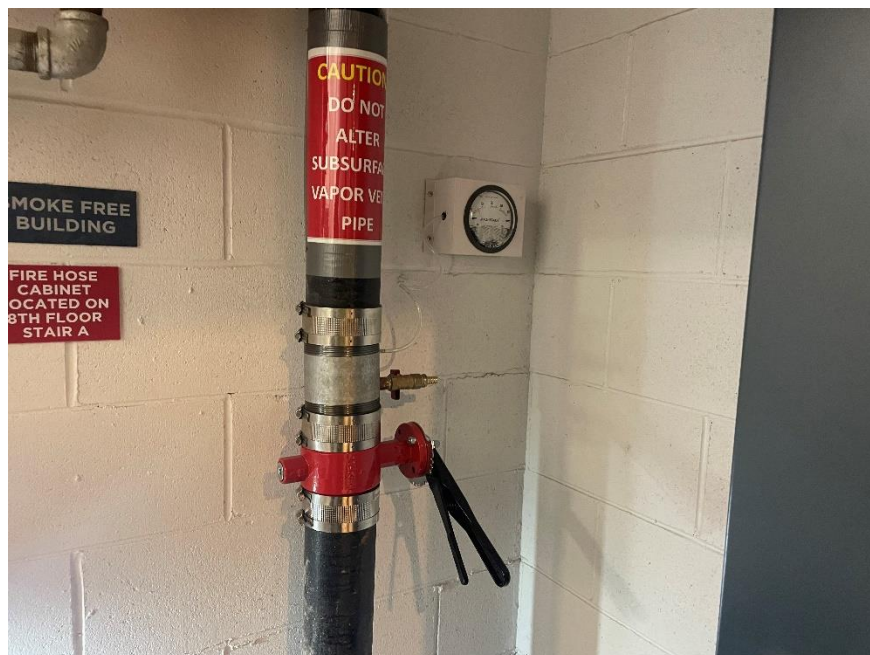
Photo 4: View of sub-membrane depressurization system (SMDS) riser that connects to Blower C.
