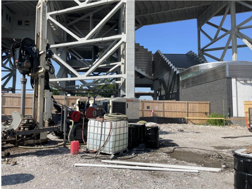
Photo 1: Geoprobe 8150LS® advancing soil boring location SB21 (facing southeast)
