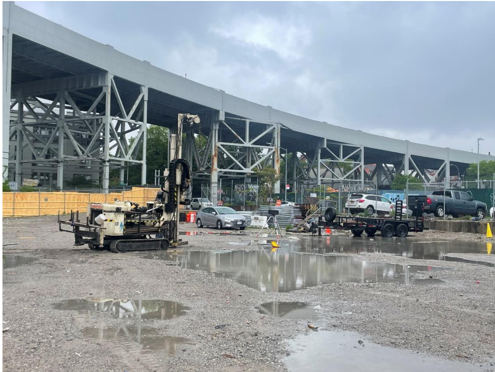
Photo 1: Geoprobe 6610DT® at GW20 location (facing northwest)
