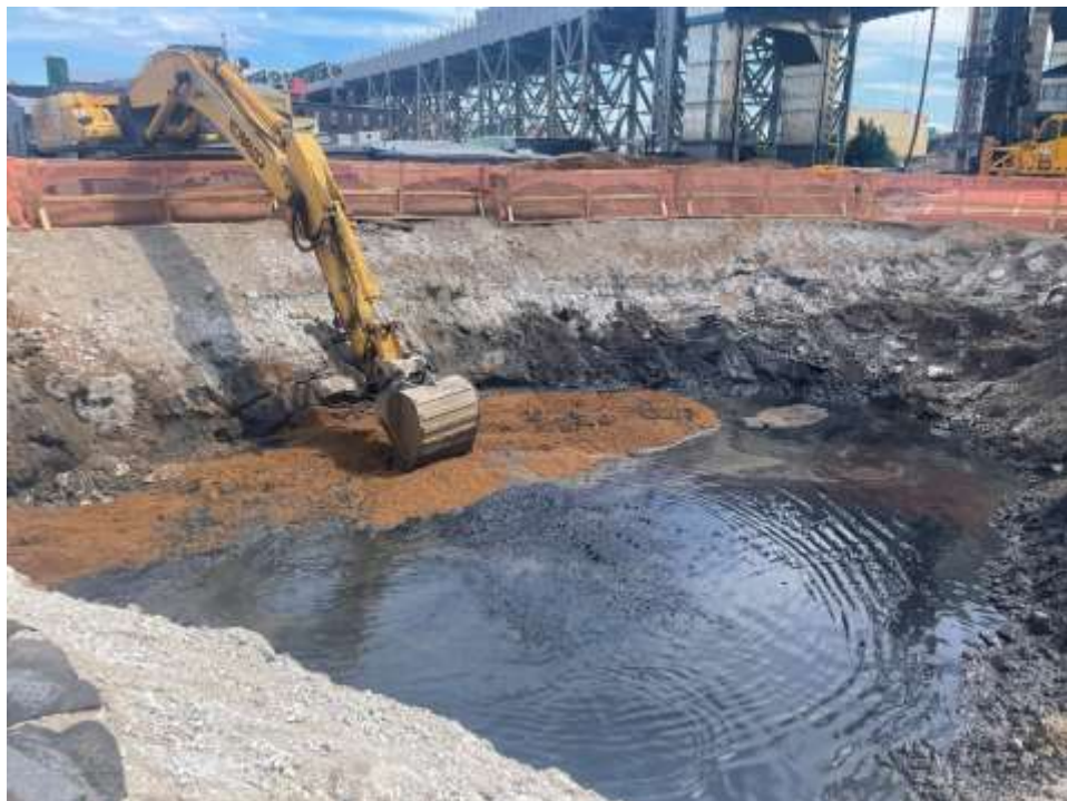
Photo 2: Bauer backfilling and mixing CSB soil into the PetroFix at the groundwater table (facing southeast).
