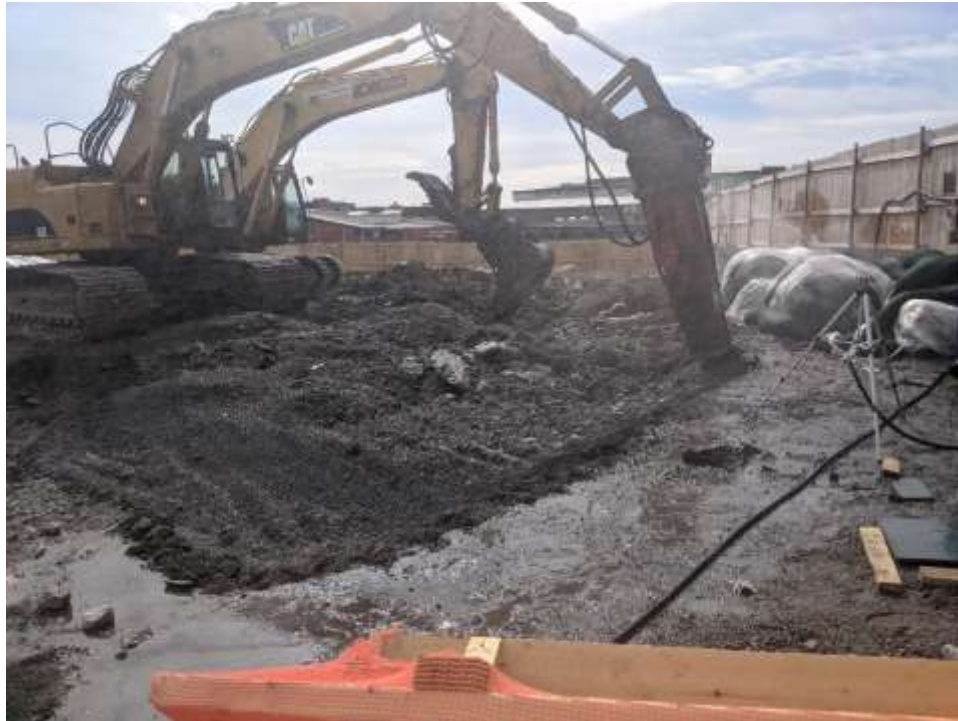
Photo 1: Bauer jackhammering and excavating concrete in the southern part of the site (facing east).
