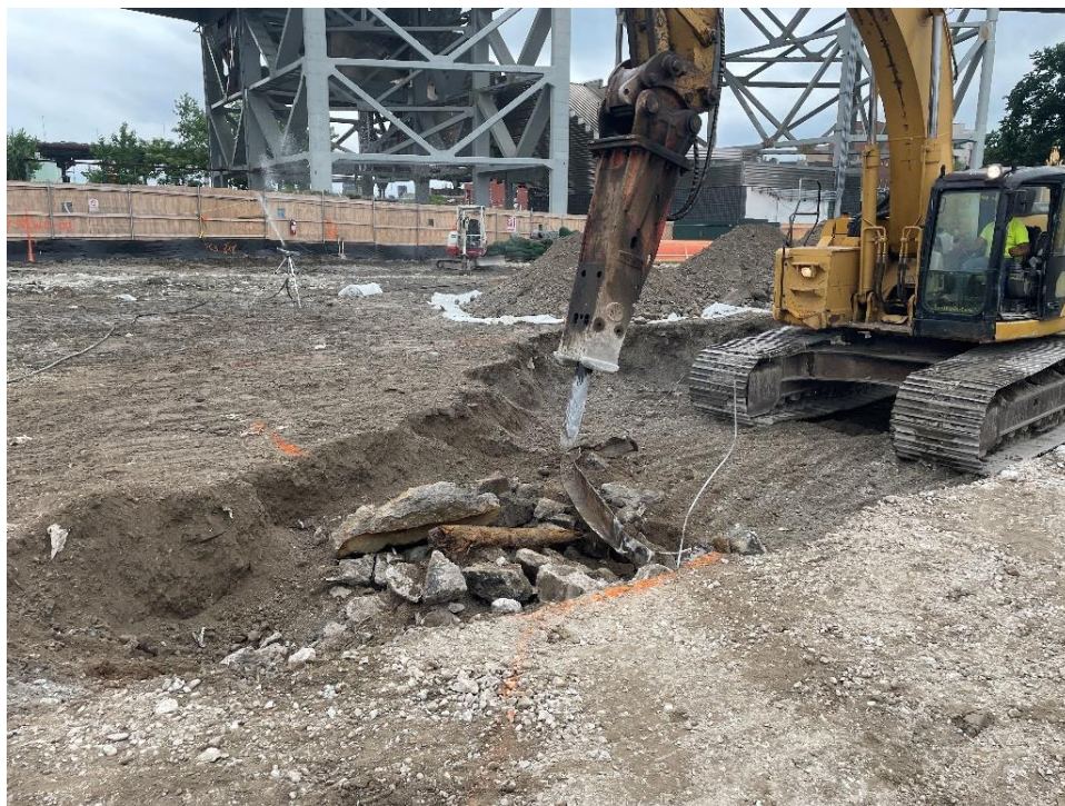
Photo 2: Bauer breaking up concrete in the central portion of the site (facing south).
