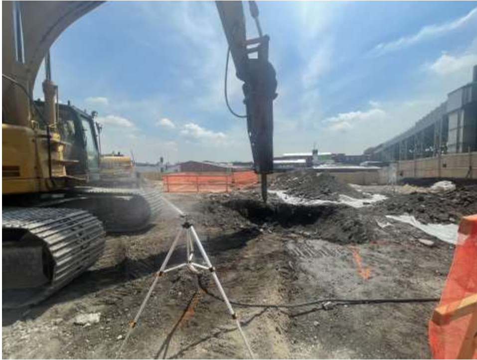
Photo 1: Bauer jackhammering and excavating concrete in the southern part of the site with sprinkler dust control (facing east).
