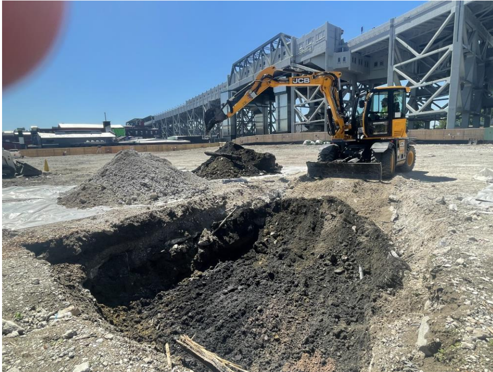
Photo 1: Bauer excavating in the northwestern portion of the site with stockpiles on polyethylene sheeting (facing southeast)
