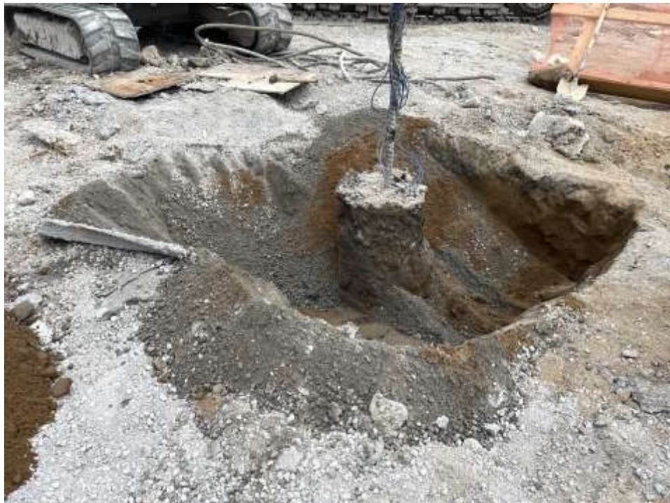
Photo 2: Morris-Shea excavating an area in the southeastern part of the site to inspect foundation piles in preparation for load testing (facing down).
