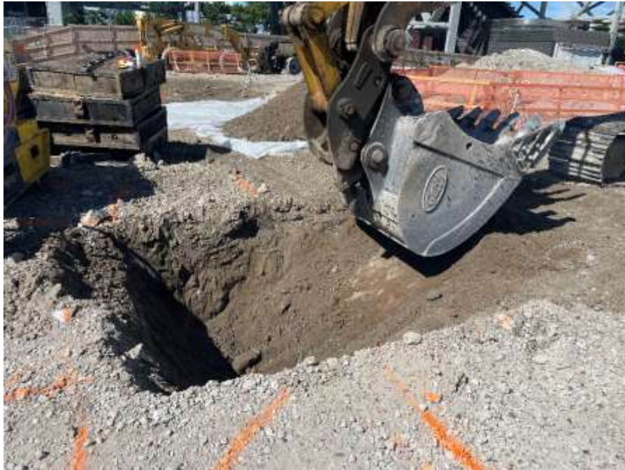
Photo 1: Bauer excavating an area in the southern portion of the site to pre-clear for obstructions. (facing south).
