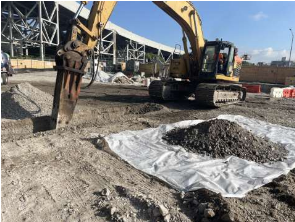
Photo 2: Bauer jackhammering an area in the central part of the site as part of waste characterization (facing northwest).
