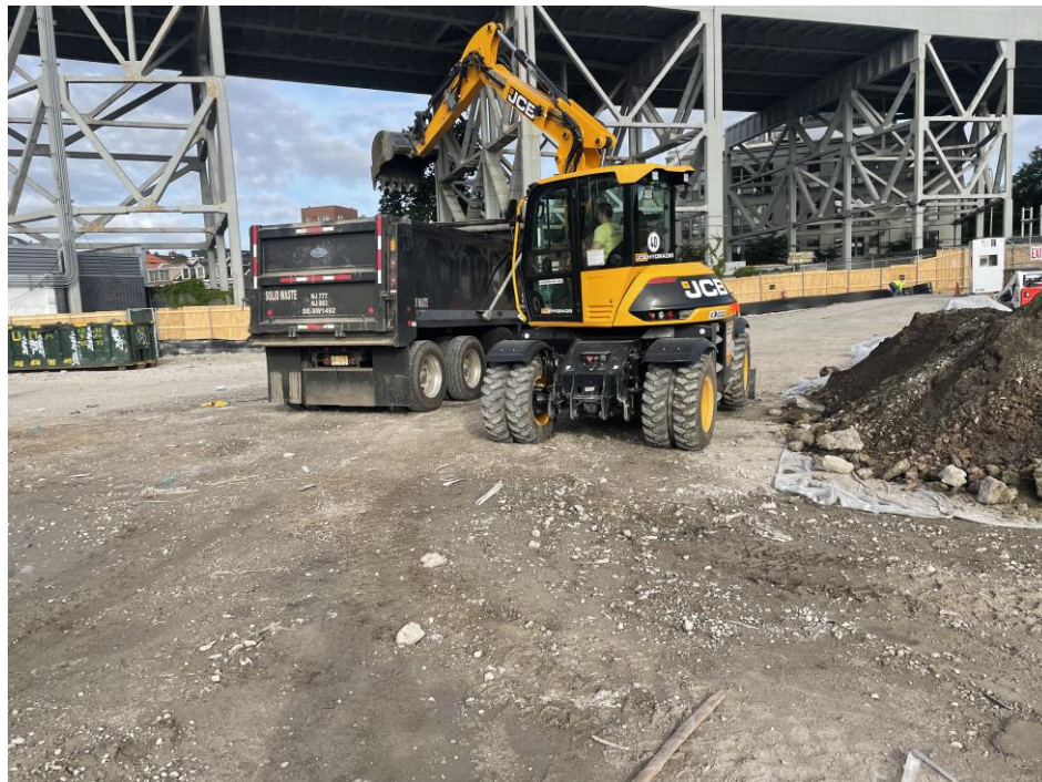
Photo 2: Bauer loading non-hazardous soil from WC05 for offsite disposal (facing west).
