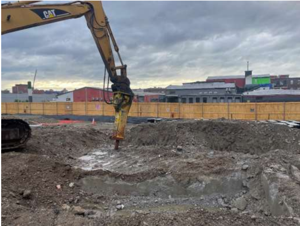
Photo 1: Bauer using a jackhammer to remove concrete in the southeastern part of the site (facing east).
