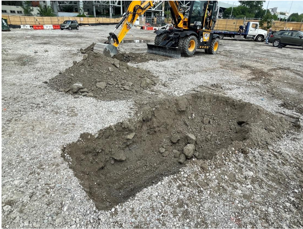
Photo 1: Bauer excavating test pits to identify concrete in preparation for pile driving (facing northwest)
