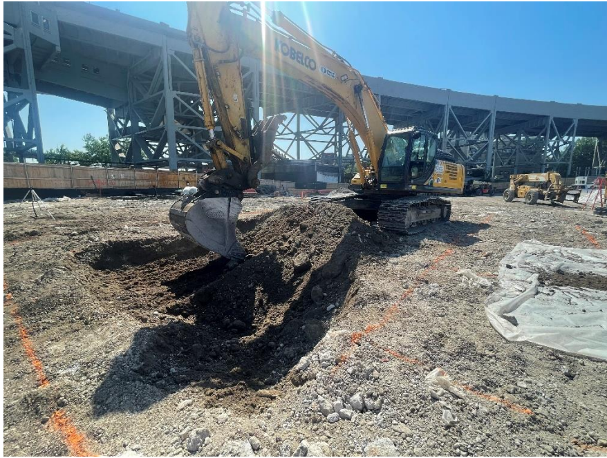
Photo 1: Bauer excavating concrete and historic fill to pre-clear concrete in the southern part of the site (facing southwest)
