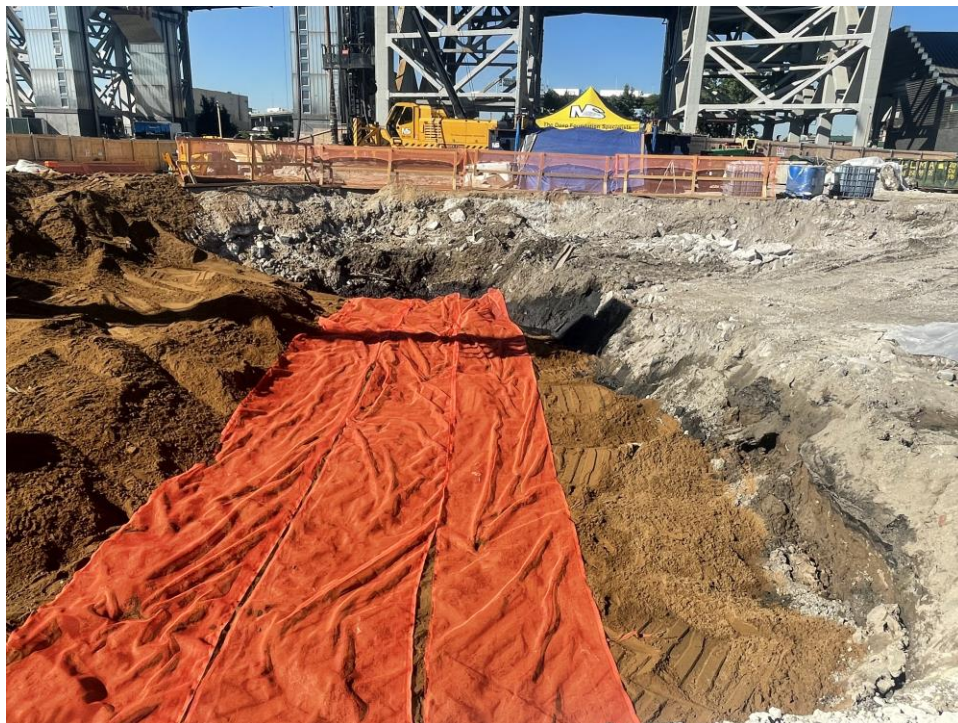
Photo 2: Bauer placed a demarcation layer at 9 feet bgs in the western part of the excavation (facing southeast).
