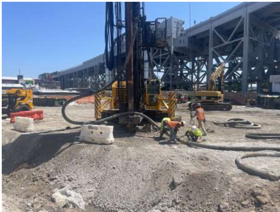
Photo 2: Morris-Shea advancing a probe pile in the northwestern area of the site (facing southeast).
