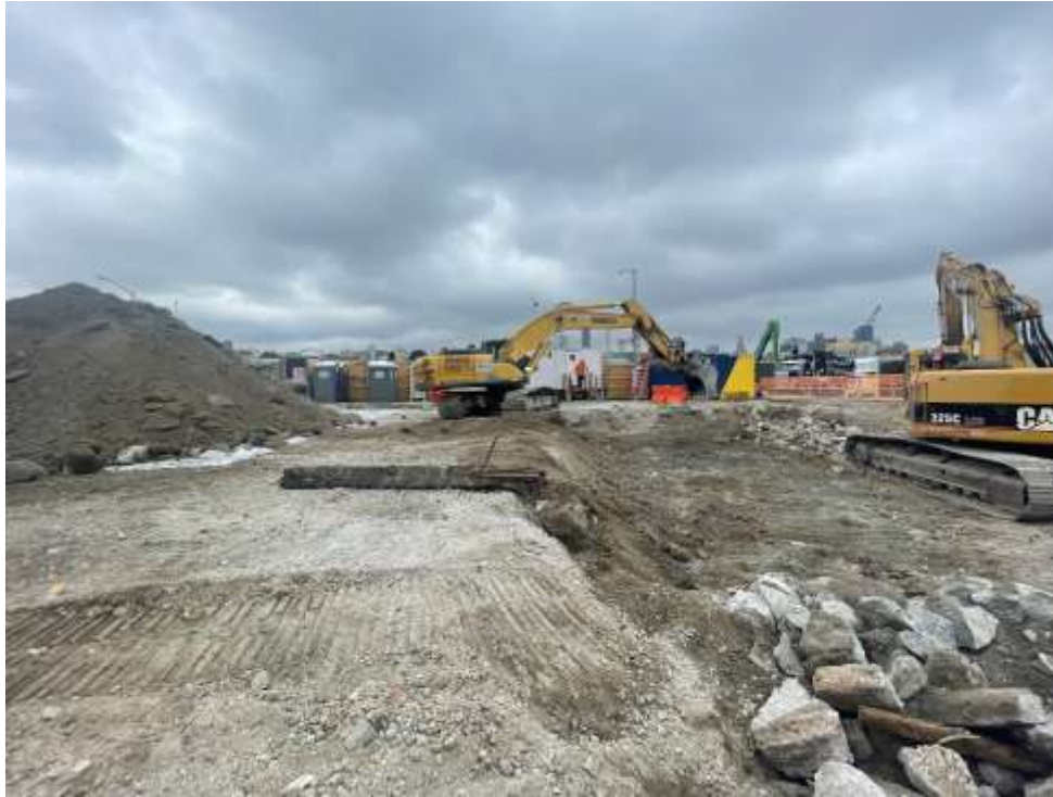
Photo 1: Bauer excavating an area in the northeastern portion of the site as part of the remedial excavation and to pre-clear for obstructions (facing northeast).
