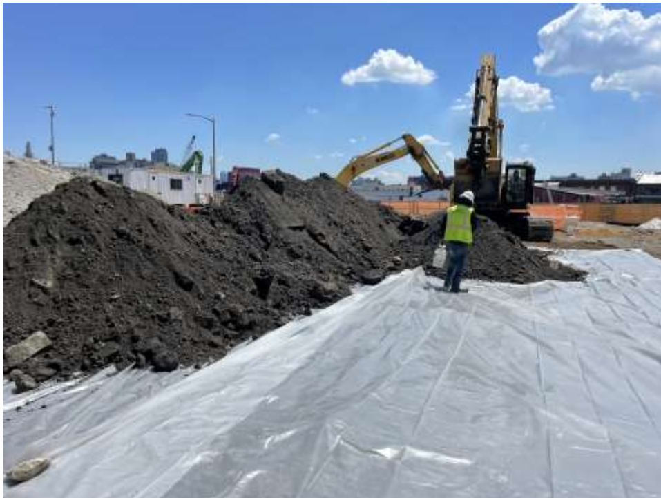
Photo 2: Bauer stockpiling excavated soil in the northeastern part of the site and applying odor suppressant prior to covering with polyethylene sheeting (facing east).
