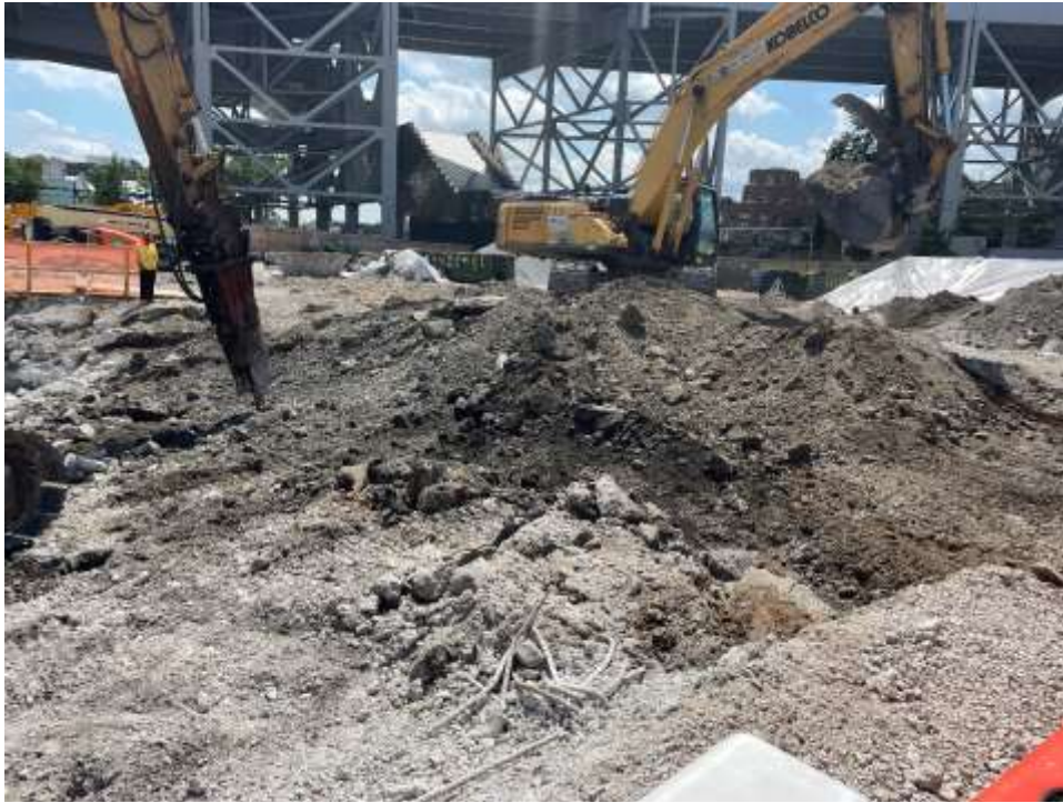
Photo 1: Bauer jackhammering an area in the central-northern portion of the site as part of the remedial excavation and to pre-clear for obstructions (facing south).
