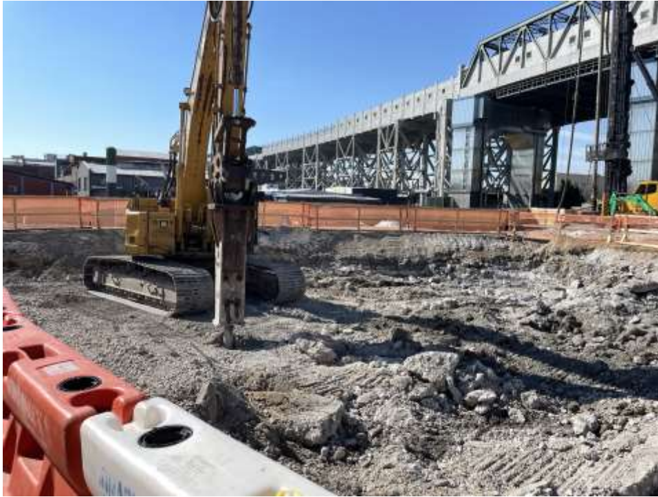
Photo 1: Bauer jackhammering an area in the central-northern portion of the site as part of the remedial excavation and to pre-clear for obstructions (facing east).
