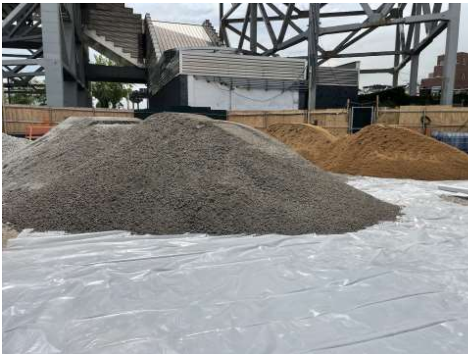
Photo 2: Bauer stockpiling imported materials on polyethylene sheeting (facing south).
