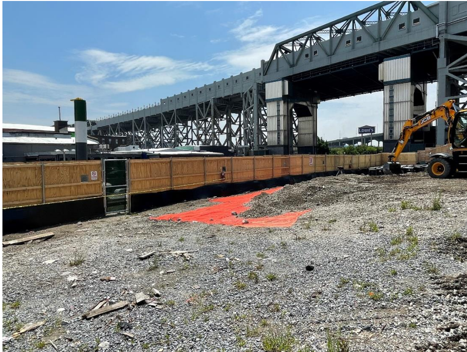
Photo 1: Crushed concrete placed over snow fencing demarcation layer along the southeastern portion of the site (facing east).
