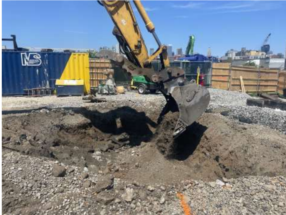
Photo 1: Bauer excavating an area in the southern portion of the site to pre-clear for obstructions (facing north).
