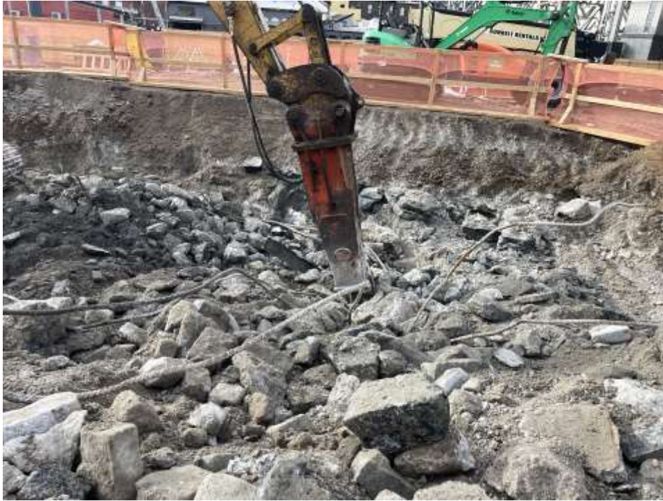
Photo 1: Bauer jackhammering an area in the eastern portion of the site as part of the remedial excavation and to pre-clear for obstructions (facing south).
