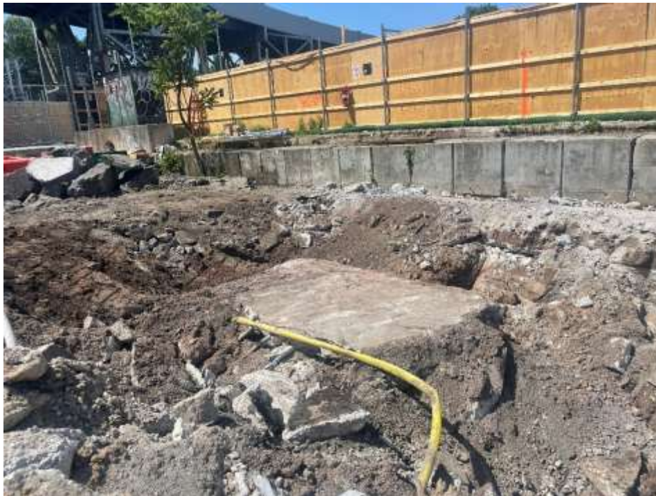
Photo 1: Concrete enclosed UST in the northwestern area of the site (facing northwest).
