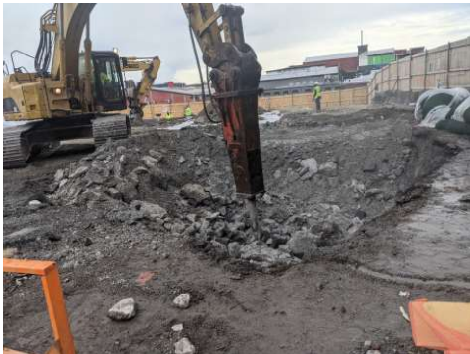
Photo 2: Bauer jackhammering concrete in the southern part of the site (facing east).
