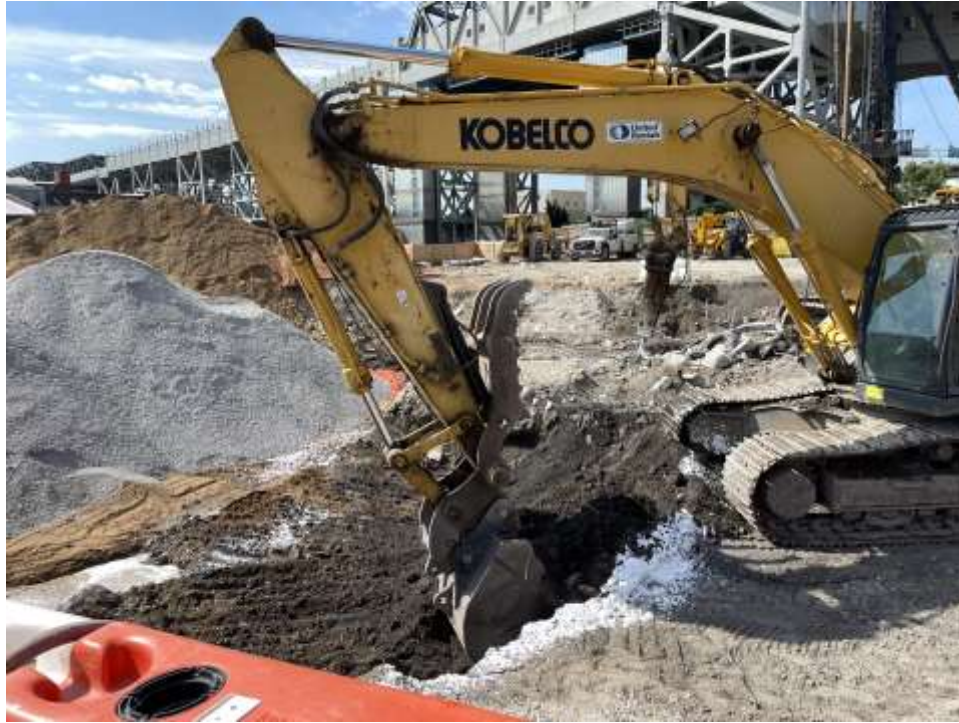
Photo 1: Bauer excavating in the northern part of the site (facing southeast).
