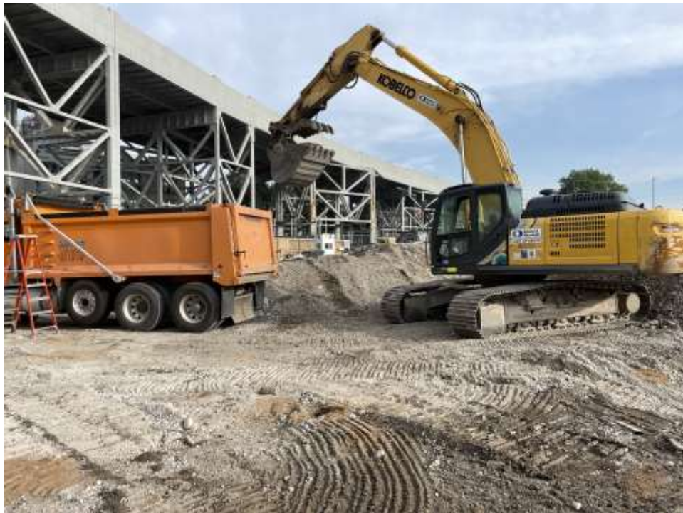
Photo 2: Bauer exporting a truckload of non-hazardous soil from grid WC08 (0-5) in the central-northern part of the site to the Clean Earth of Carteret facility located in Carteret, New Jersey (facing north).
