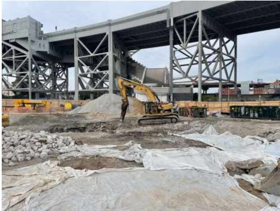
Photo 1: Bauer jackhammering in the central part of the site (facing southwest).
