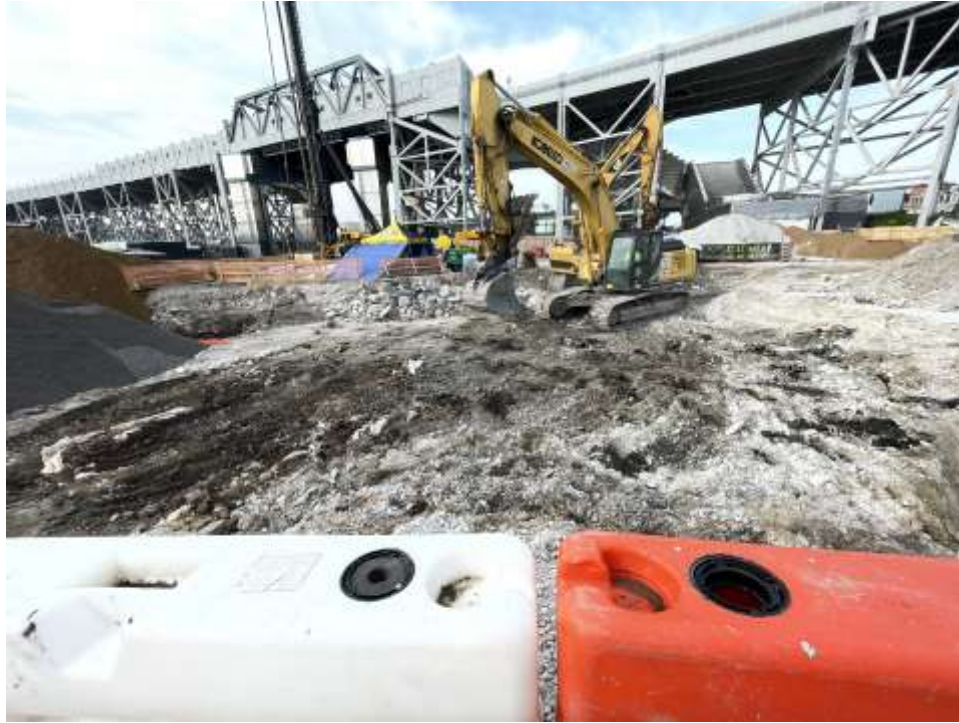
Photo 1: Bauer excavating in the central-northern part of the site (facing south).
