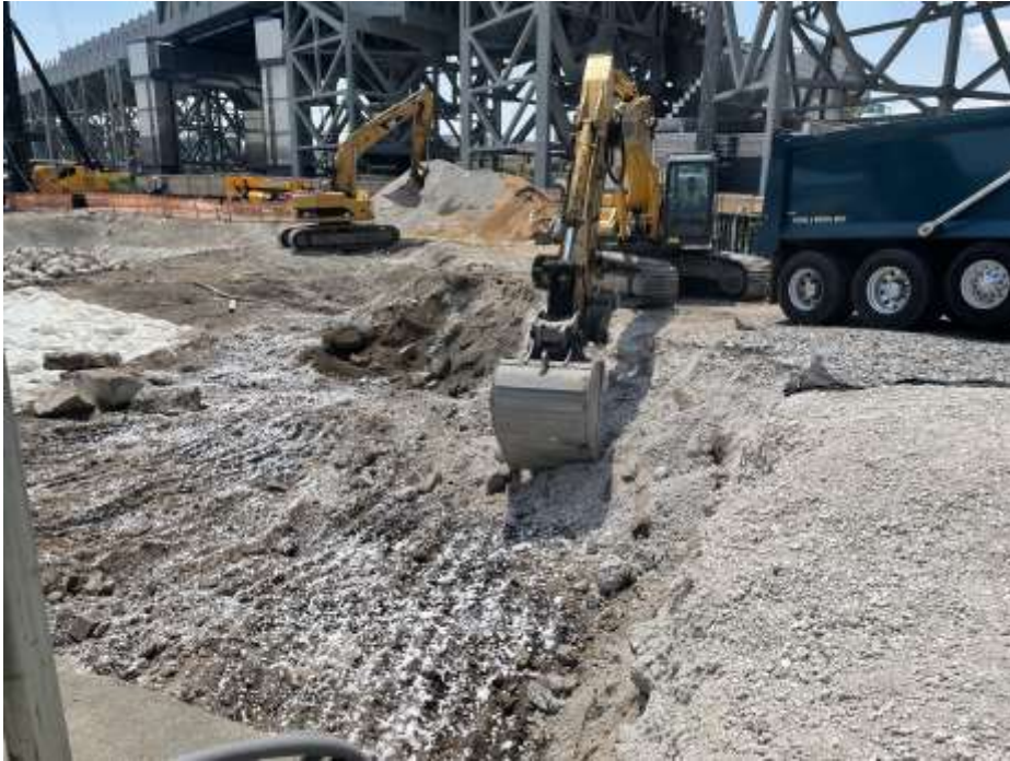
Photo 1: Bauer excavating in the northwestern part of the site (facing southeast).
