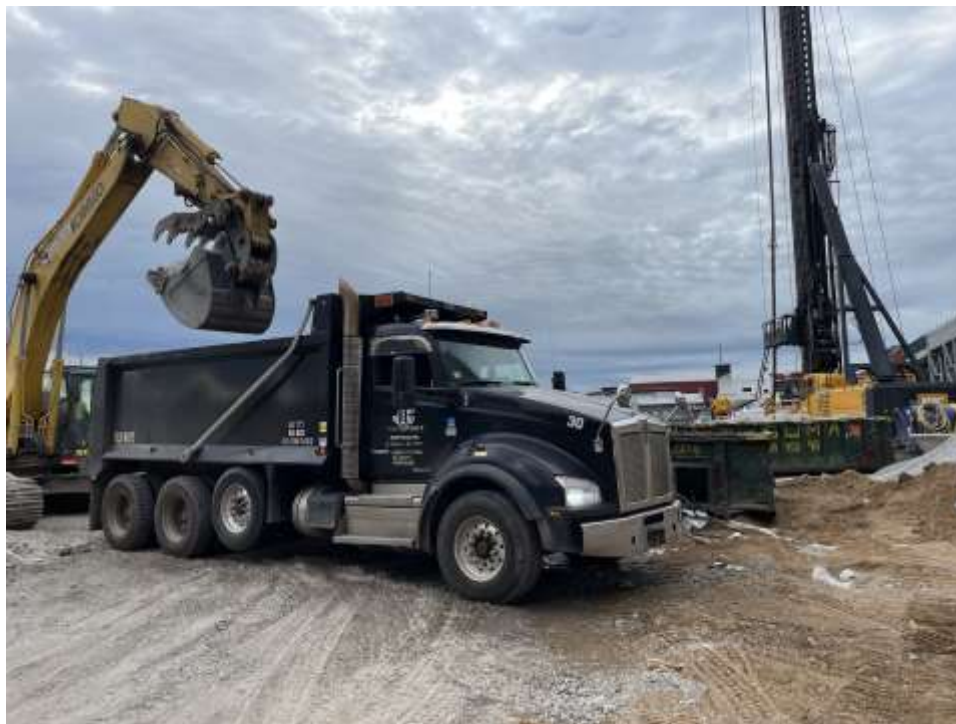
Photo 2: Bauer exporting a truckload of non-hazardous soil from grid WC08 (0-5) in the central-northern part of the site to the Clean Earth of Carteret facility located in Carteret, New Jersey (facing east).
