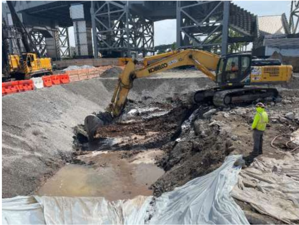
Photo 1: Bauer excavating in the northern area of the site (facing south).
