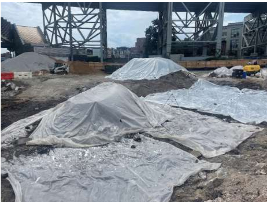
Photo 2: Poly sheeting covering inactive stockpiles across the site (facing south).
