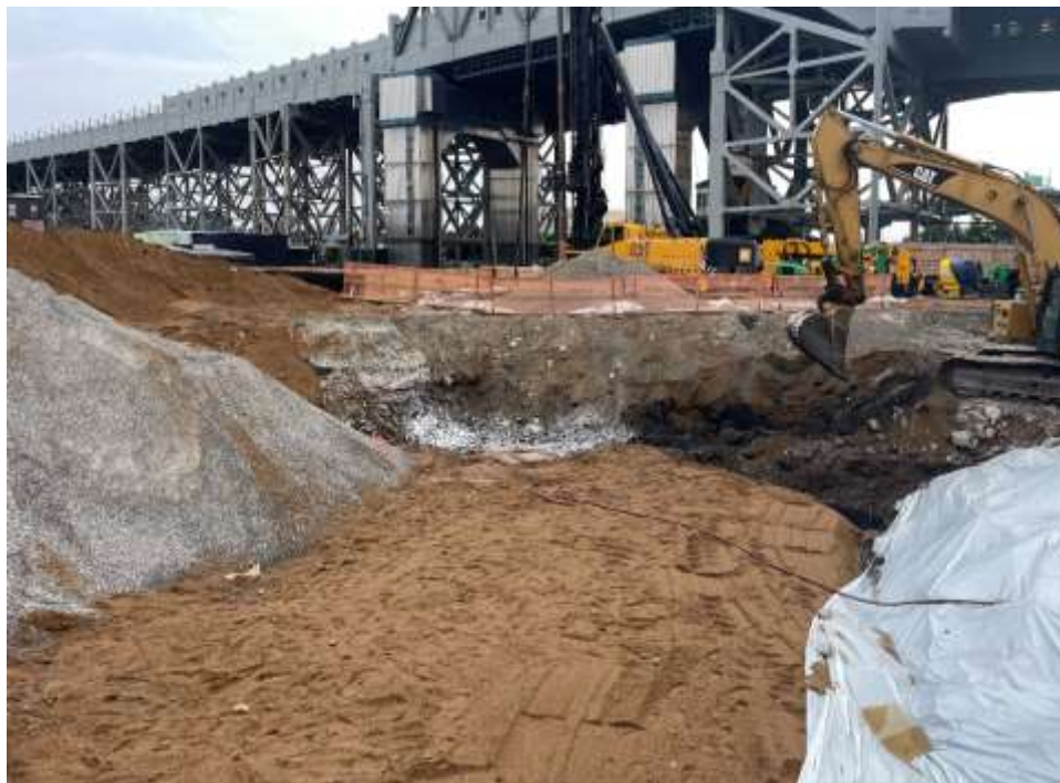
Photo 2: Bauer excavating in the central part of the site (facing south).
