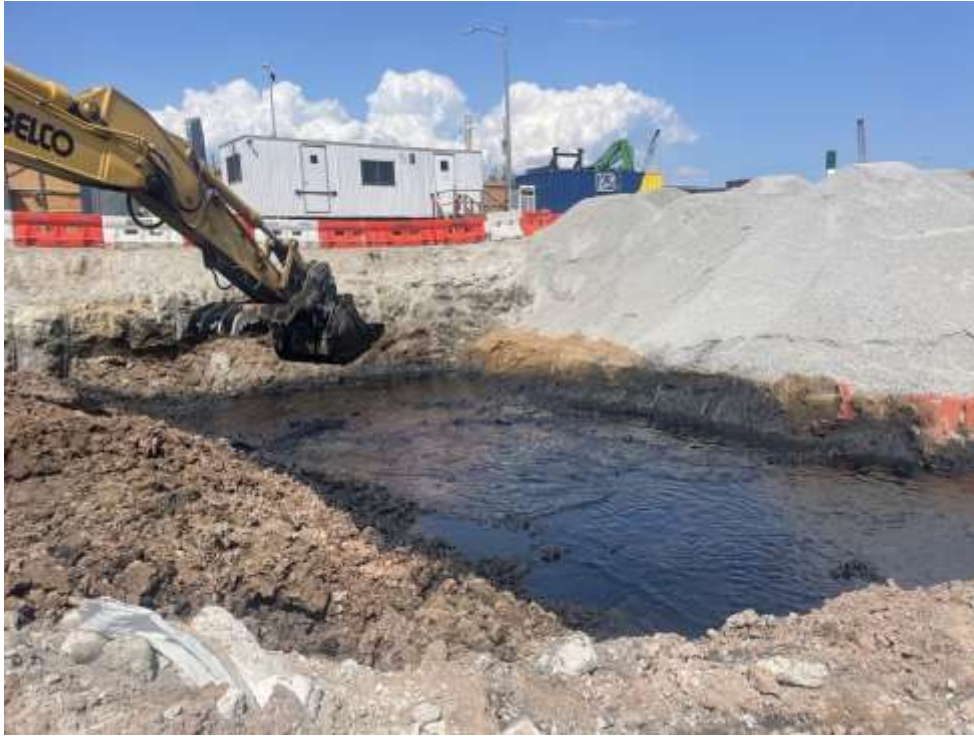
Photo 1: PetroFix application in the northeastern area of the site (facing northeast).
