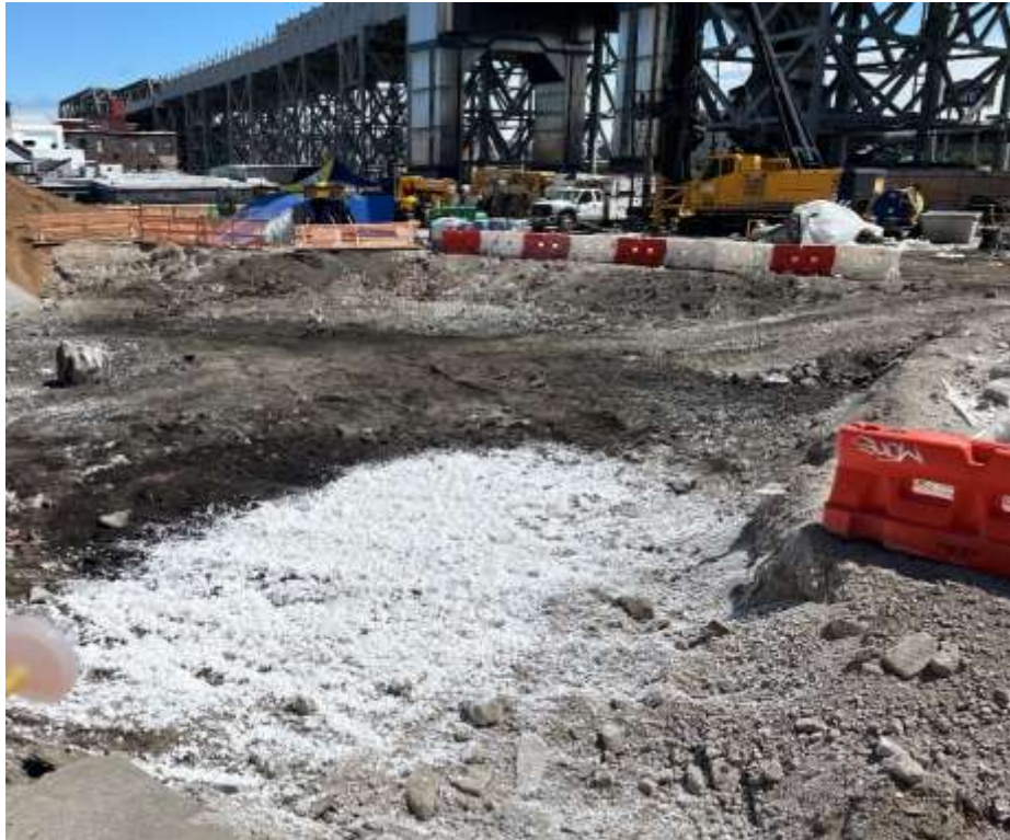
Photo 1: Bauer applying odor-suppressing foam to the bottom of excavation (facing south).
