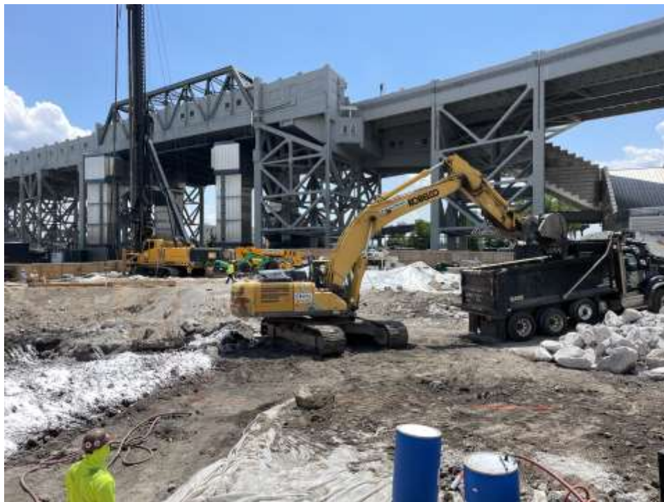
Photo 2: Bauer loading a tri-axle truck with non-hazardous soil for offsite disposal (facing south).
