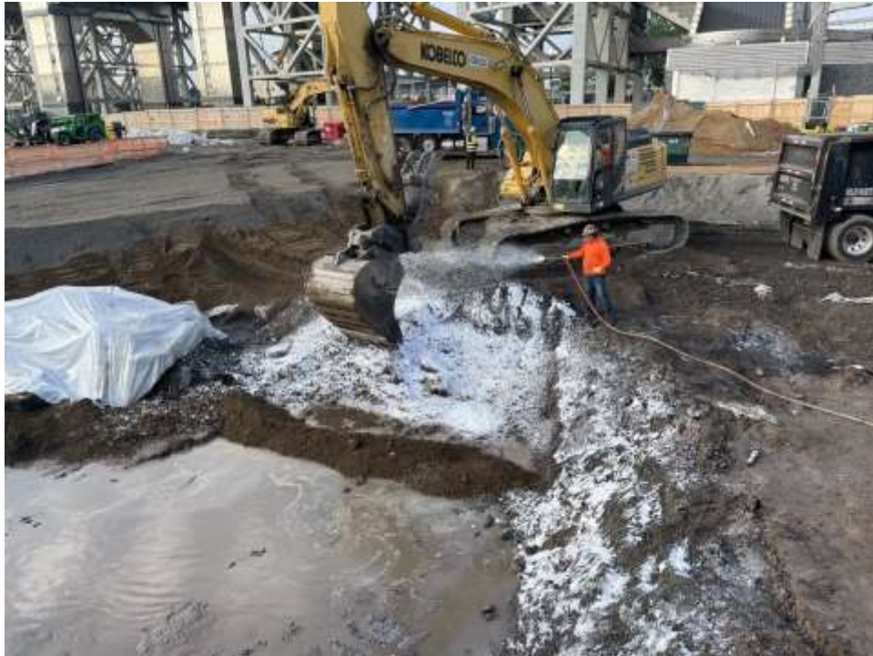
Photo 1: Bauer applying odor suppressing foam to the excavation area in the northern part of the site (facing south).
