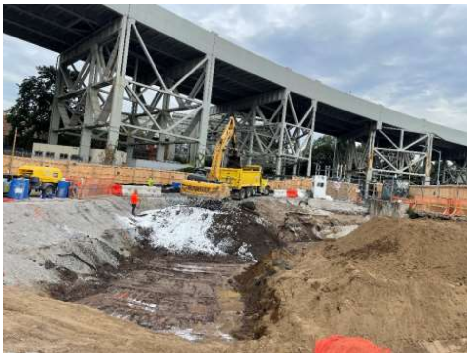
Photo 1: Bauer applying odor suppressing foam to the excavation area in the northwestern part of the site (facing west).
