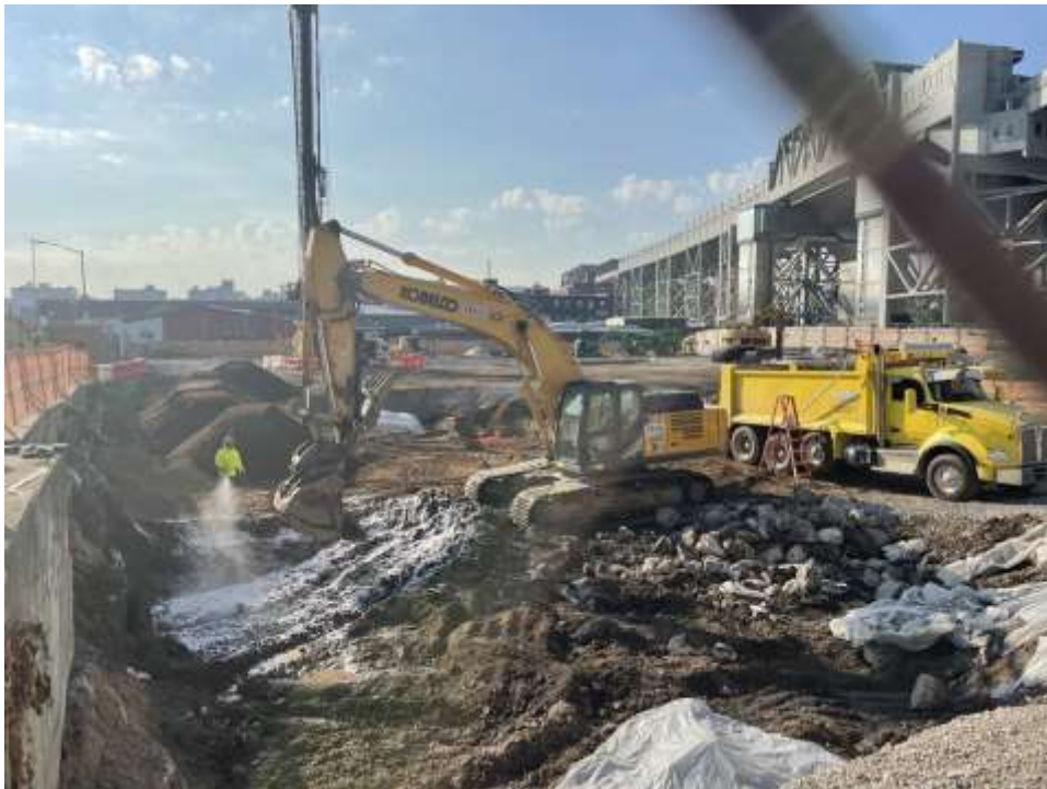
Photo 2: Bauer excavating and using odor suppressing foam in the northwestern part of the site (facing east).
