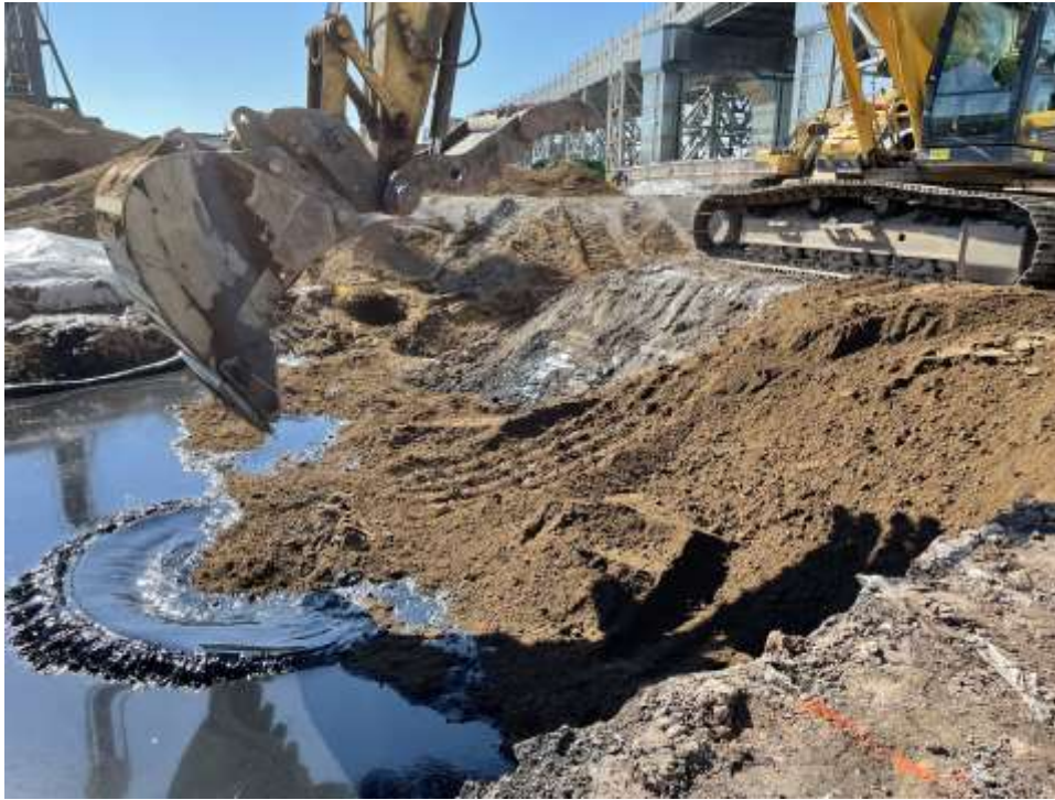
Photo 1: Bauer mixing clean fill into groundwater with PetroFix™ at the base of the excavation area in the northern part of the site (facing south).
