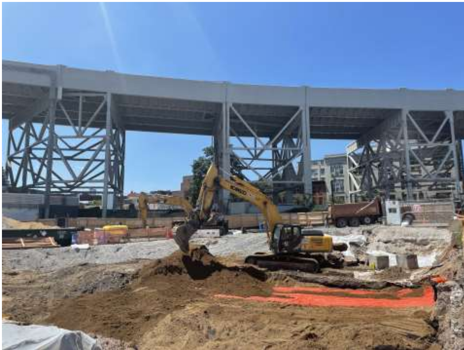
Photo 2: Bauer backfilling and placing orange snow fence as a demarcation barrier in the northern part of the site (facing west).
