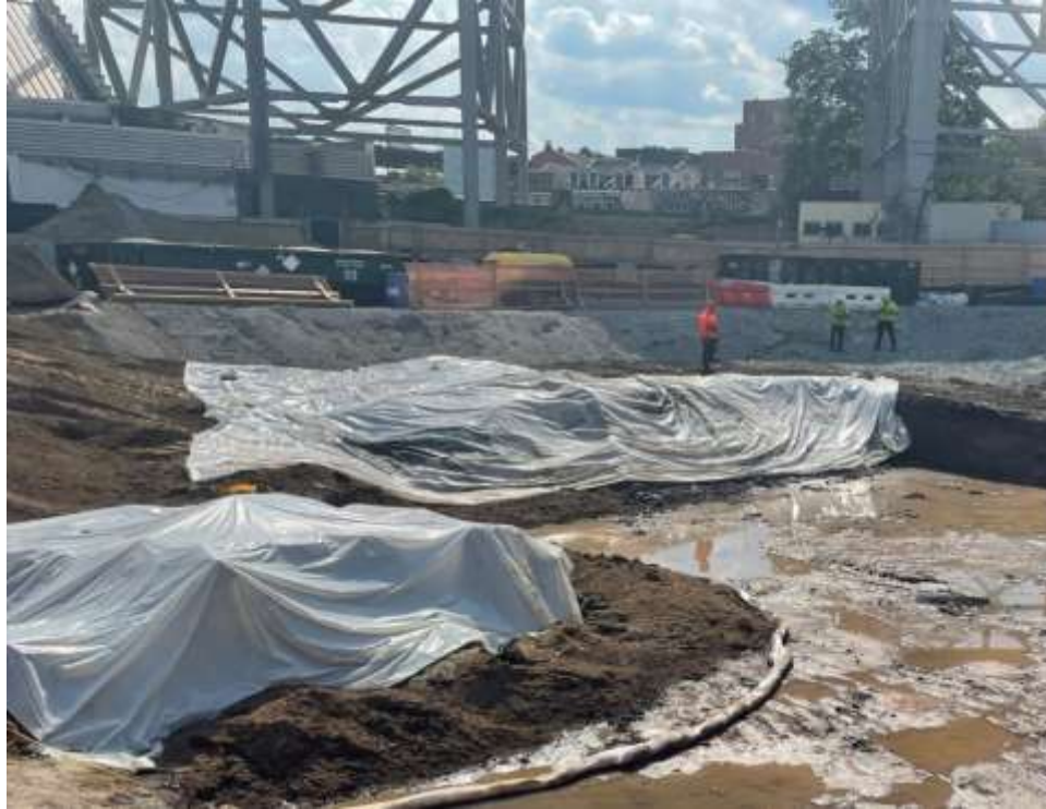
Photo 2: Bauer covering the exposed excavation area with polyethylene sheeting at the end of the day in the northern part of the site (facing southwest).
