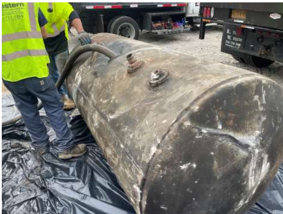
Photo 2: Eastern vacuuming the contents of one UST (facing northwest).
