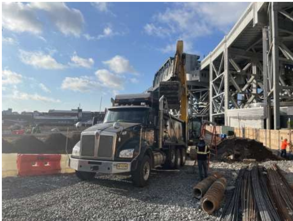
Photo 1: Bauer loading soil for export to Clean Earth of Carteret (facing southeast).
