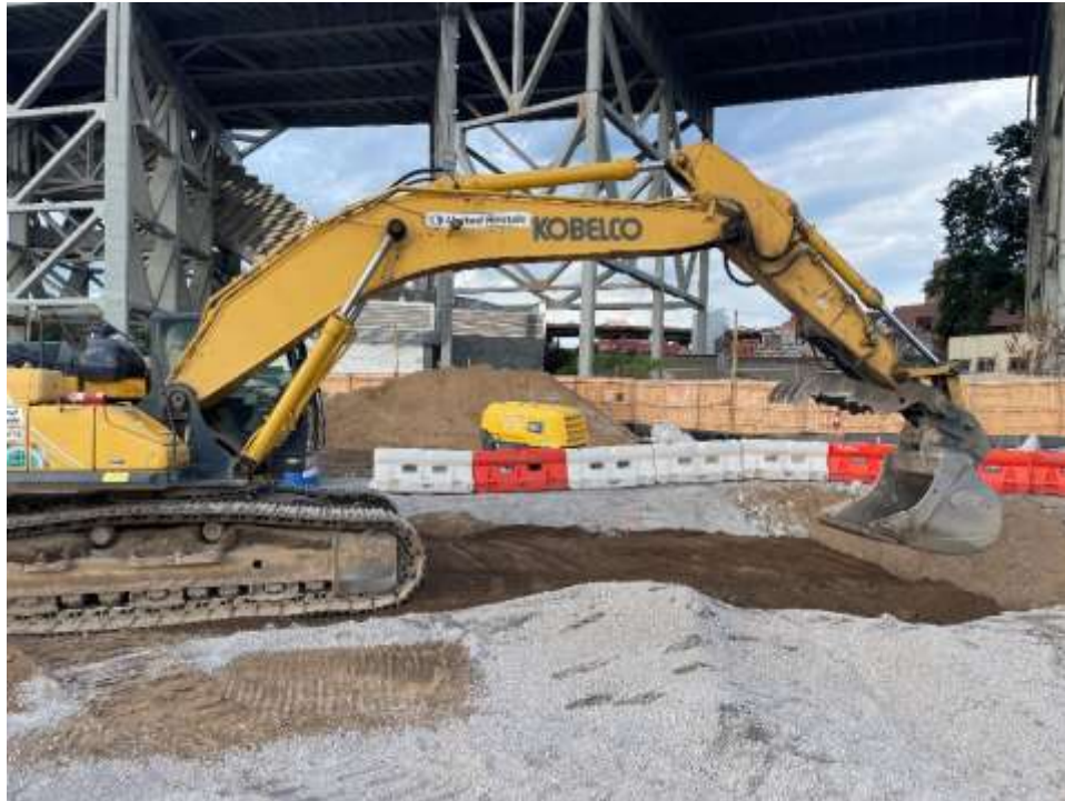
Photo 1: Bauer backfilling an area in the western part of the site with imported clean fill from Evergreen Recycling of Corona (facing south).
