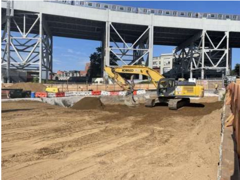
Photo 1: Bauer backfilling an area in the western part of the site with imported clean fill from EROC (facing southwest).
