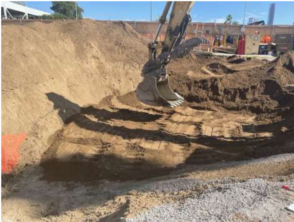
Photo 2: Bauer backfilling an area with imported clean fill from EROC (facing north).
