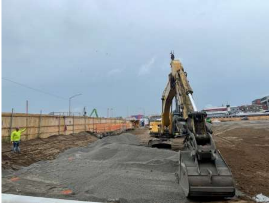
Photo 1: Bauer backfilling an area in the northwestern part of the site with RCA (facing east).
