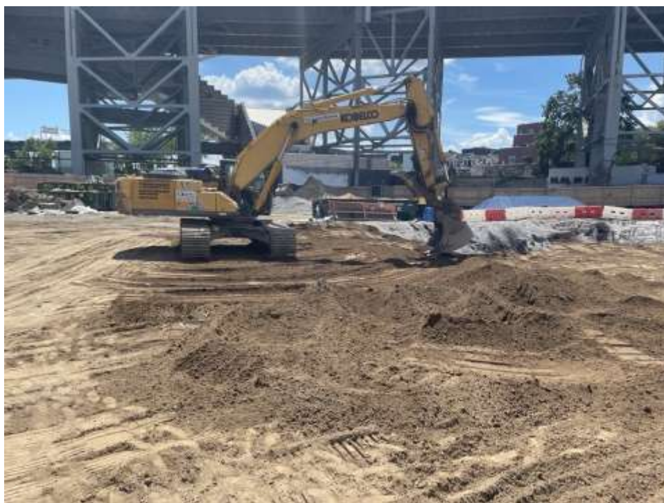
Photo 2: Bauer backfilling an area in the central part of the site with imported clean fill from EROC (facing south).
