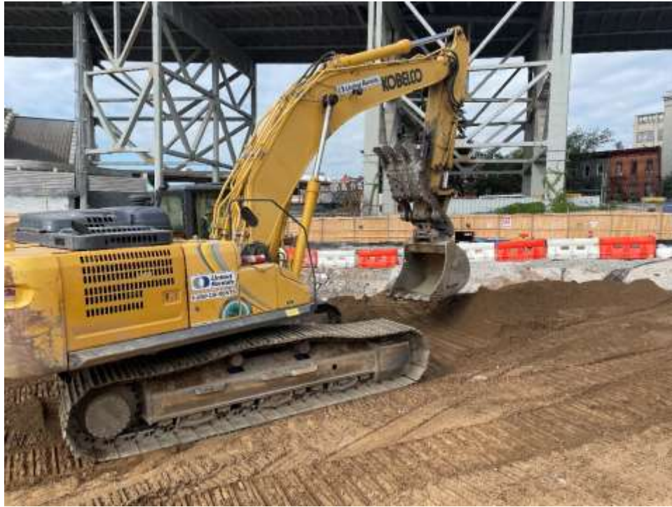
Photo 1: Bauer backfilling in the northwestern part of the site (facing southwest).
