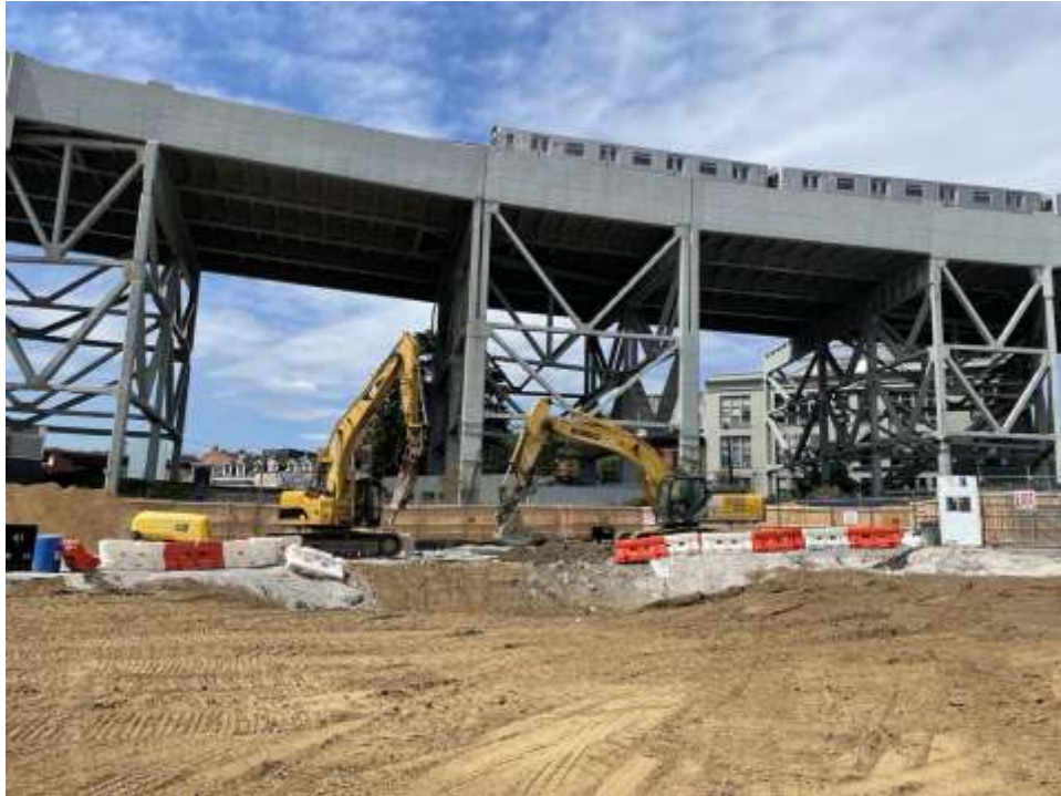
Photo 2: Bauer pre-clearing in the western part of the site (facing west).
