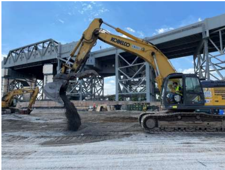
Photo 2: Bauer backfilling an area in the central part of the site with RCA (facing southeast).
