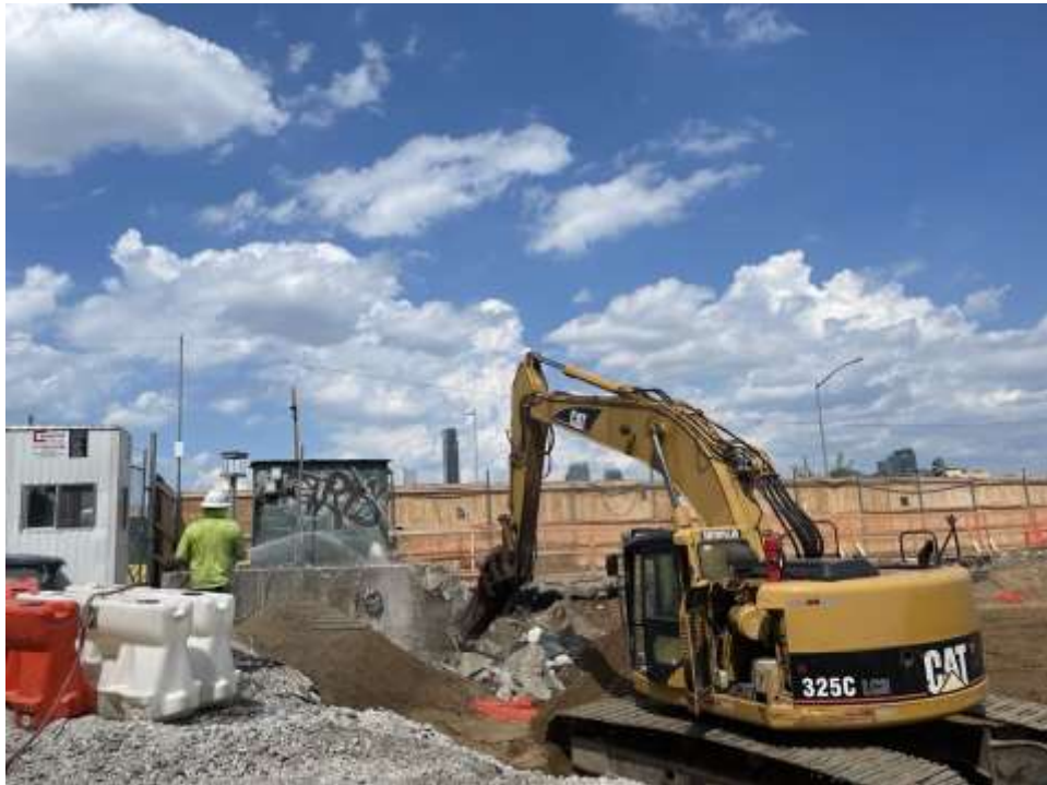
Photo 2: Bauer using dust suppression during jackhammering concrete in the northwestern part of the site (facing north).
