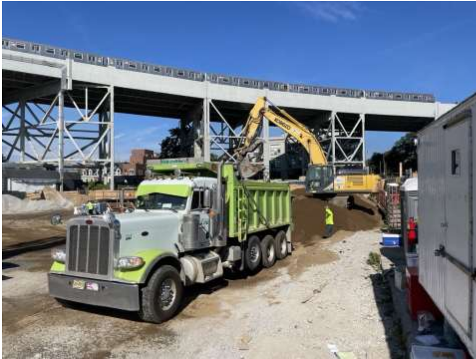
Photo 1: Bauer importing clean fill from Evergreen Recycling of Corona for backfill of the excavation areas (facing west).
