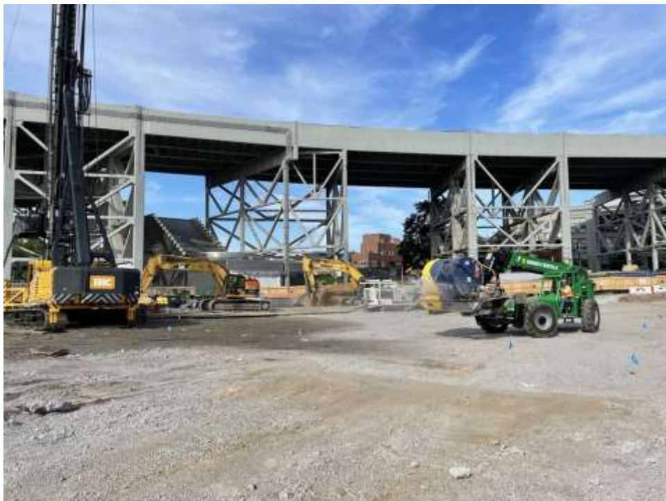
Photo 2: Morris-Shea spraying water throughout the site to mitigate dust (facing south).
