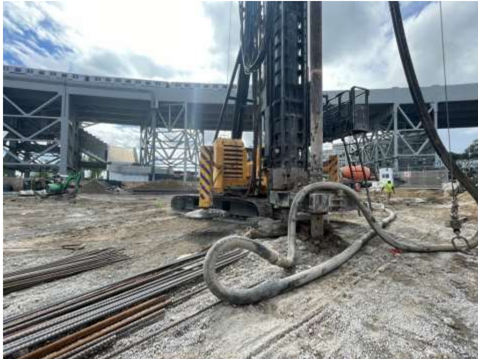
Photo 1: Morris-Shea advancing piles in the western part of the site (facing south).
