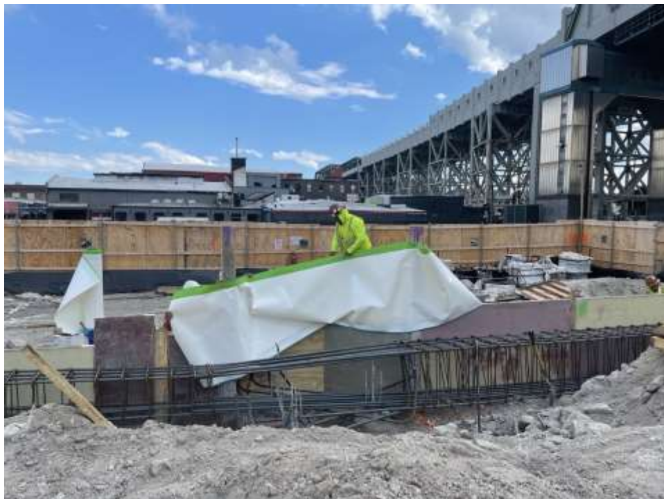
Photo 2: Bauer placing waterproofing/vapor barrier membrane (Preprufe 160R Plus) on the exterior foundation walls of the formwork (facing east).
