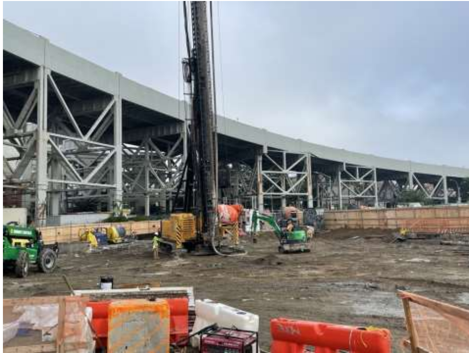
Photo 1: Morris-Shea advancing piles in the western part of the site (facing northwest).
