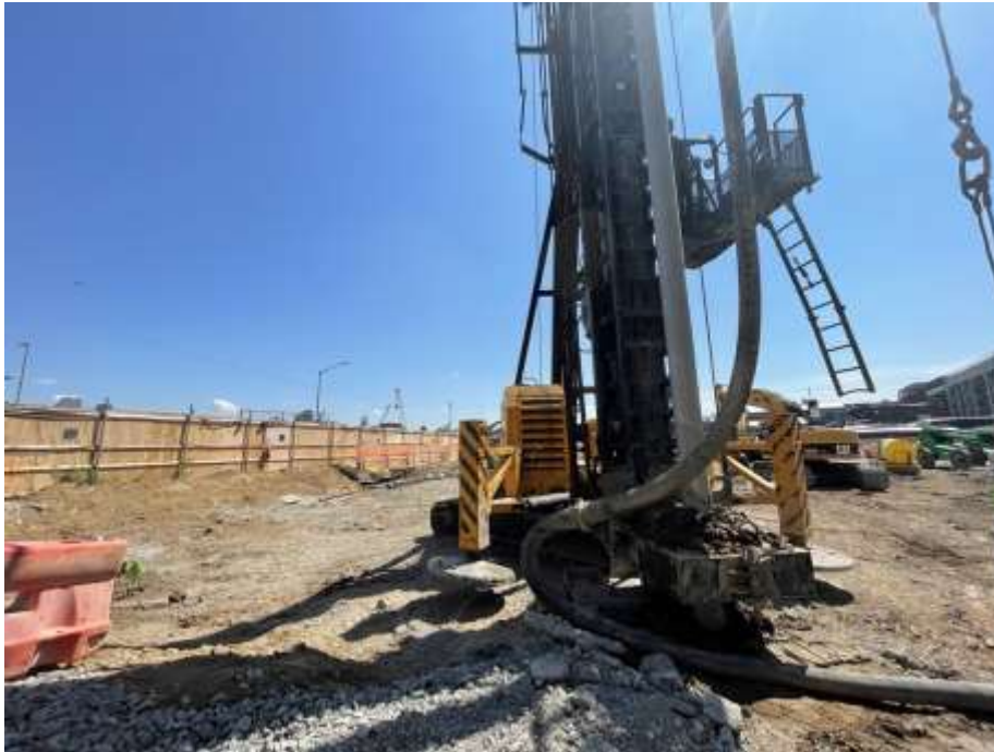
Photo 1: Morris-Shea advancing piles in the western part of the site (facing northeast).
