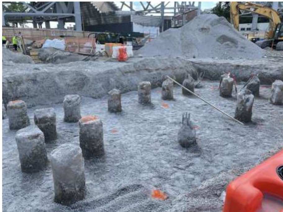
Photo 2: The excavation area in the central part of the site prepared for pile cap formwork installation (facing southwest).
