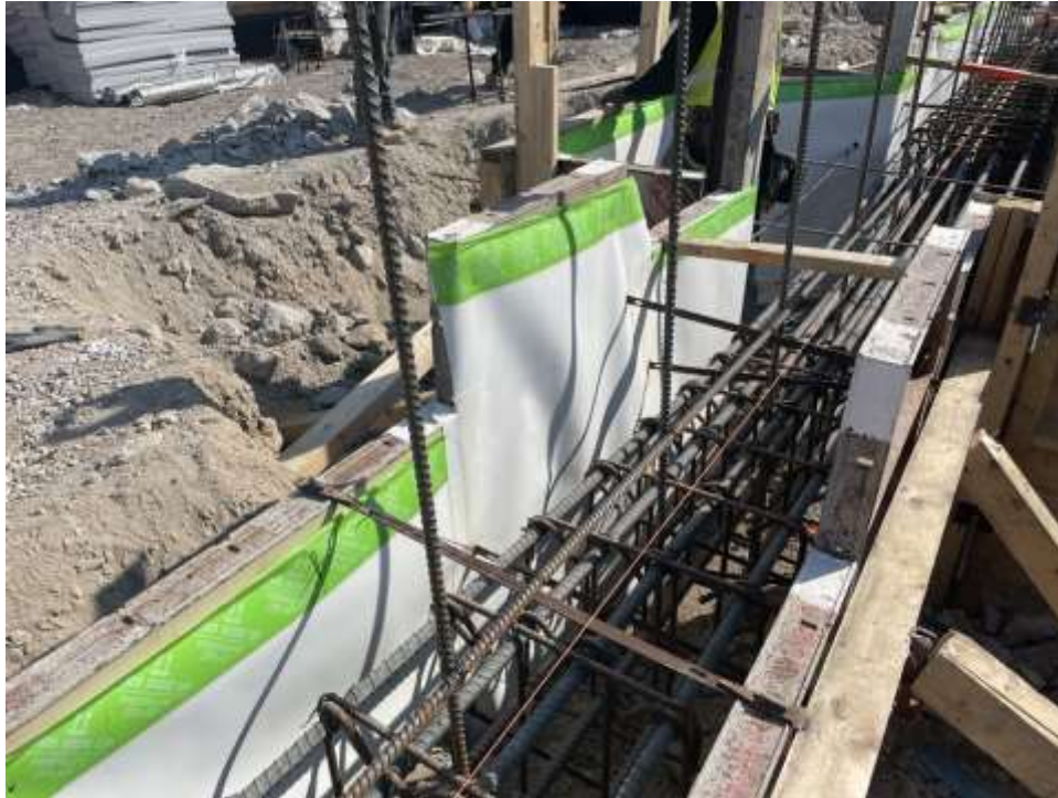
Photo 1: Bauer installing waterproofing/vapor barrier membrane (Preprufe 160R Plus) in the southeastern part of the site (facing southeast).
