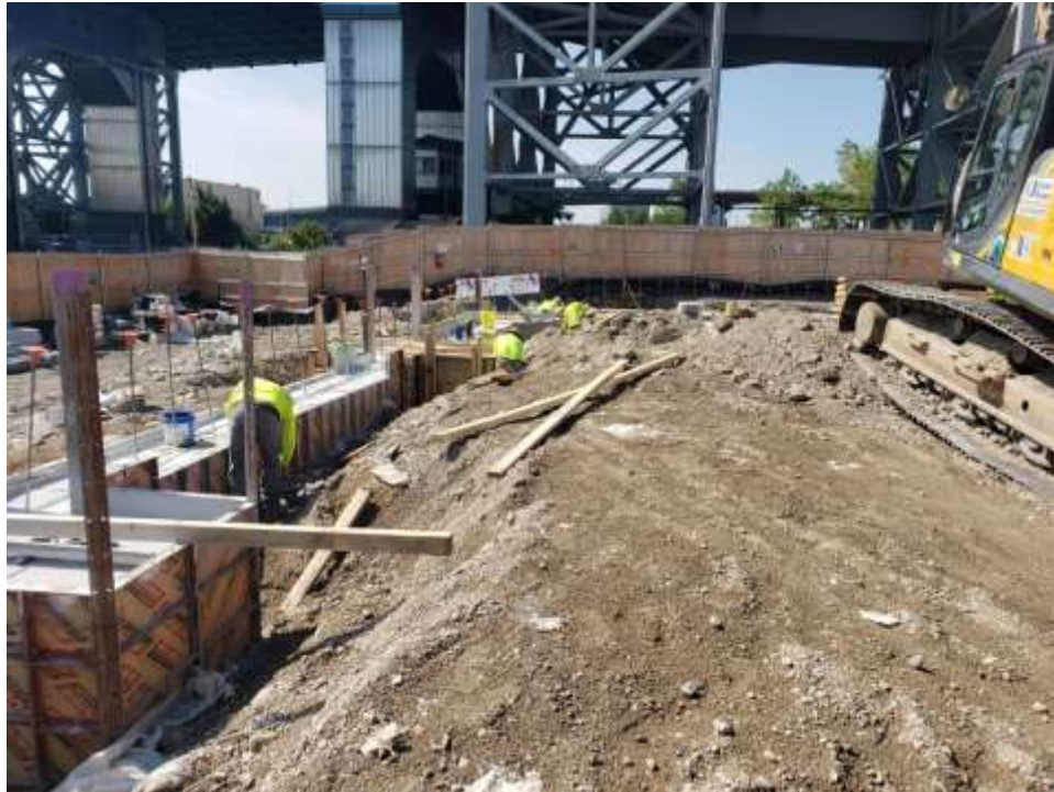
Photo 1: Bauer removing foundation formwork in the southwestern part of the site (facing southwest).
