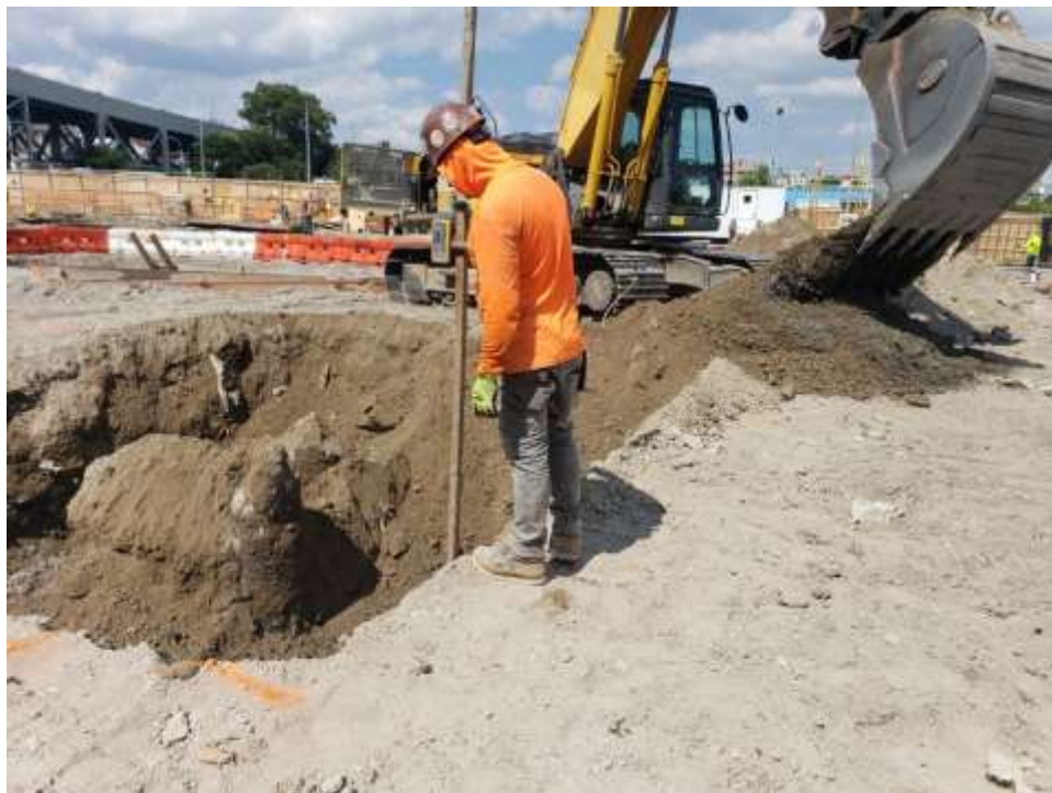
Photo 2: Bauer excavating around foundation elements in the central part of the site (facing north).
