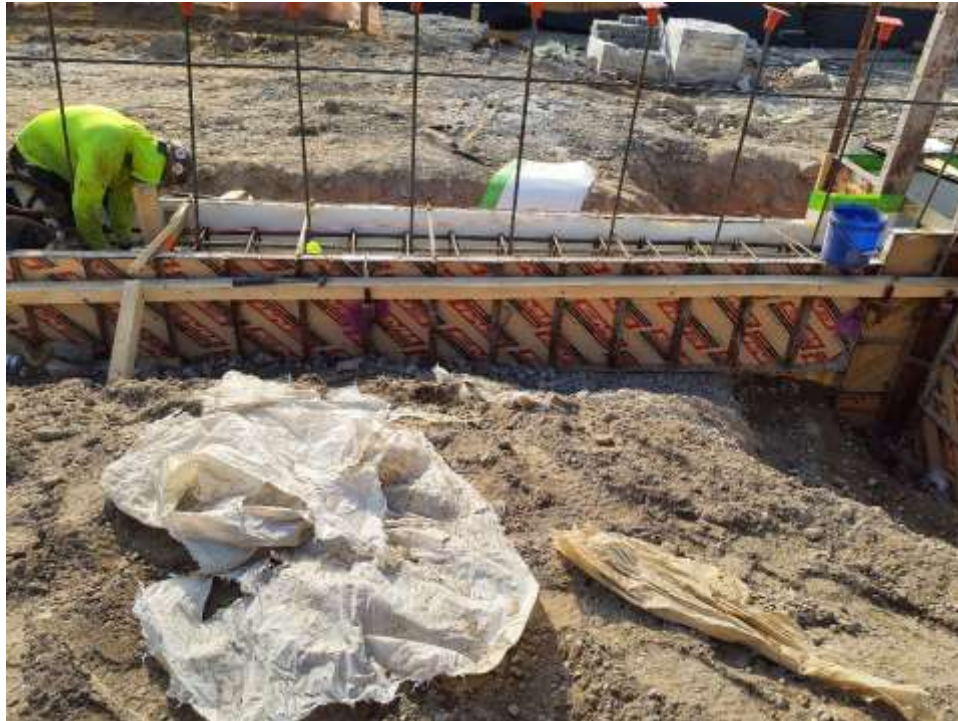
Photo 1: Bauer installing rebar in the eastern part of the site (facing east).
