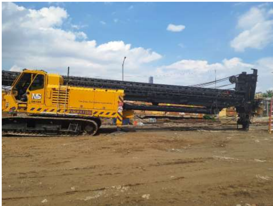
Photo 2: Morris Shea demobilizing the Fundex F2800 Drill Rig
