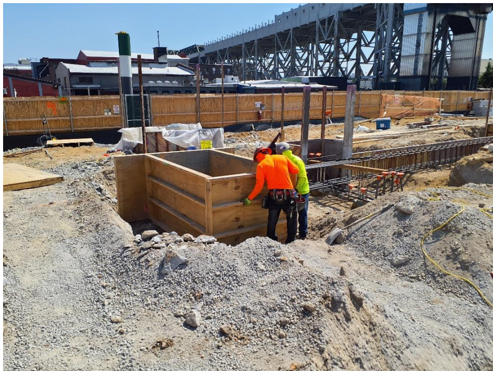
Photo 2: Bauer installing formwork in the northeastern part of the site (facing southeast).
