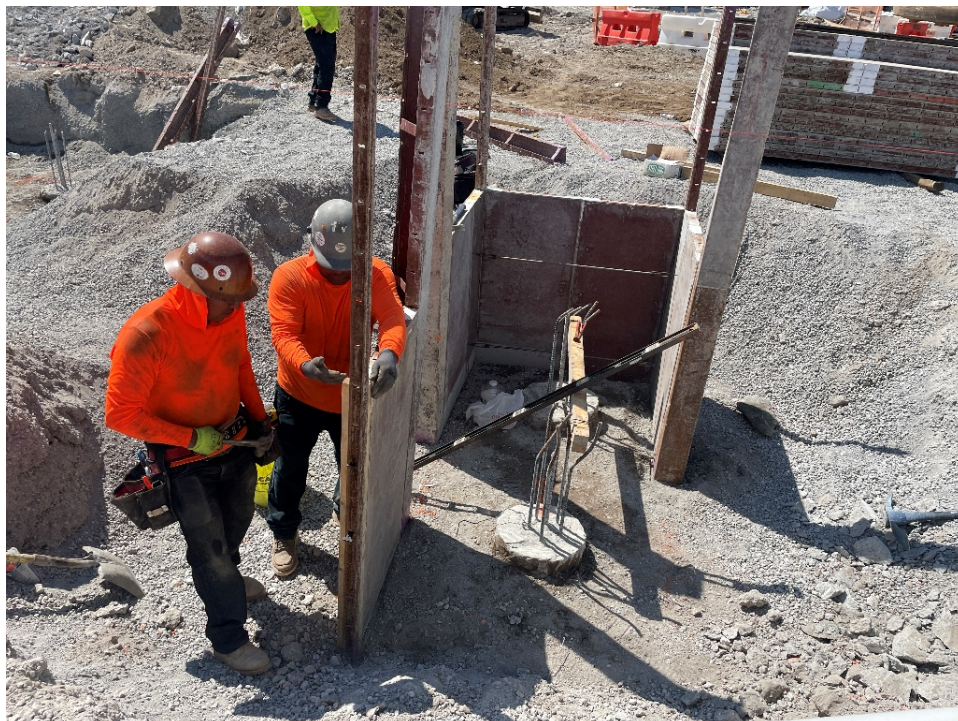
Photo 2: Bauer installing formwork in the northern part of the site (facing southeast)
