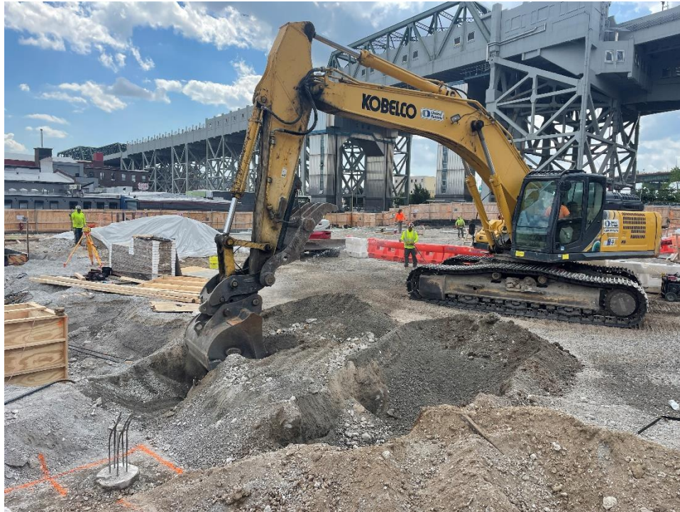
Photo 1: Bauer excavating around piles in the northeastern part of the site (facing south)
