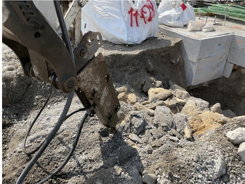
Photo 1: Bauer chopping concrete for piping installation in the southeastern part of the site (facing southwest).
