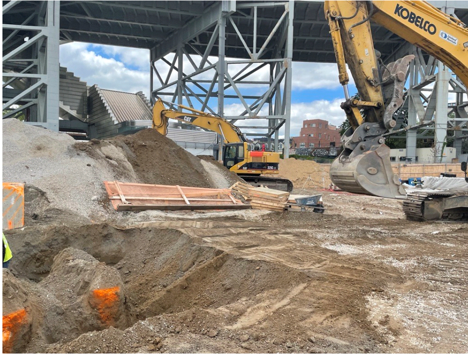
Photo 1: Bauer excavating for pile cap installation in the north-central part of the site (facing southwest).
