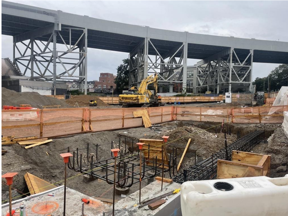
Photo 1: Bauer installing formwork in the northern part of the site (facing southwest)
