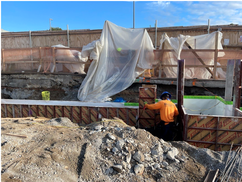
Photo 2: Bauer installing the waterproofing/vapor barrier membrane (Preprufe 160R Plus) within the formwork in the northern part of the site (facing north).
