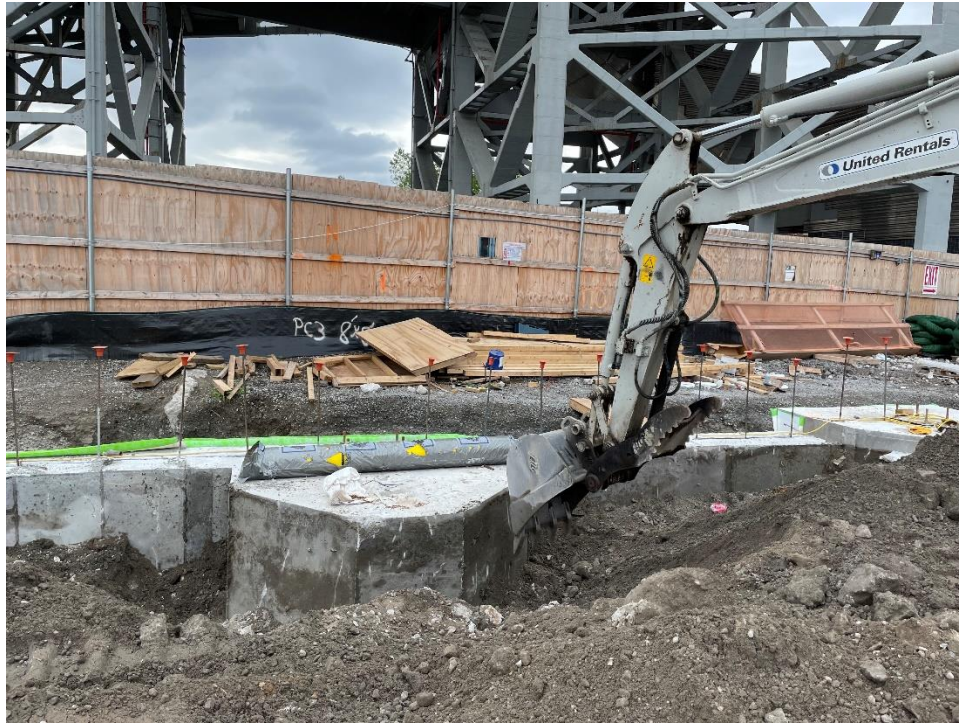
Photo 1: Bauer excavating to remove formwork in the southeastern part of the site (facing southeast).
