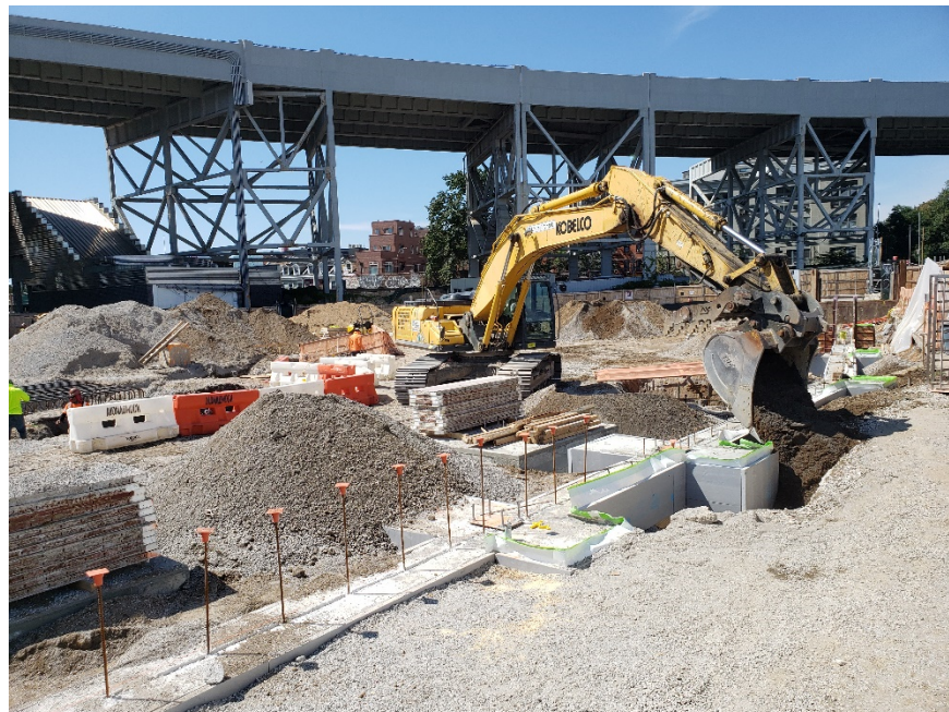
Photo 2: Bauer backfilling using previously imported clean fill and RCA in the northern part of the site (facing southwest)
