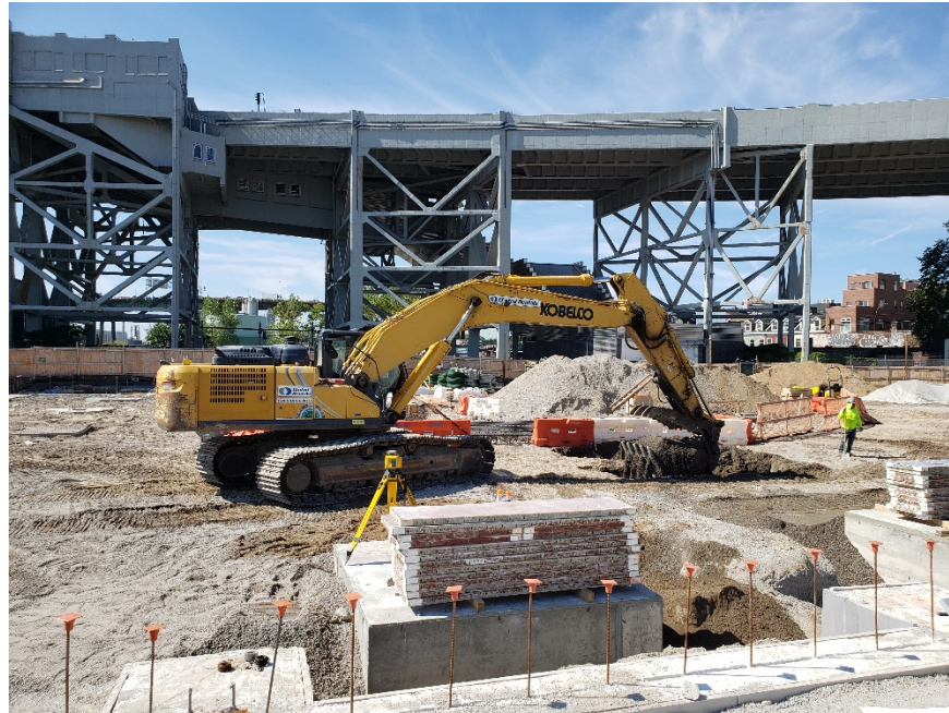
Photo 1: Bauer excavating previously imported clean fill and RCA for pile cap installation in the north-central part of the site (facing south).
