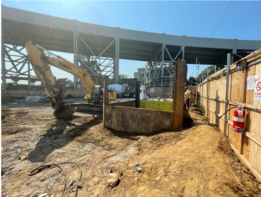
Photo 1: Bauer installing the shoring box and excavating within the shoring box in the northwestern part of the site (facing west).
