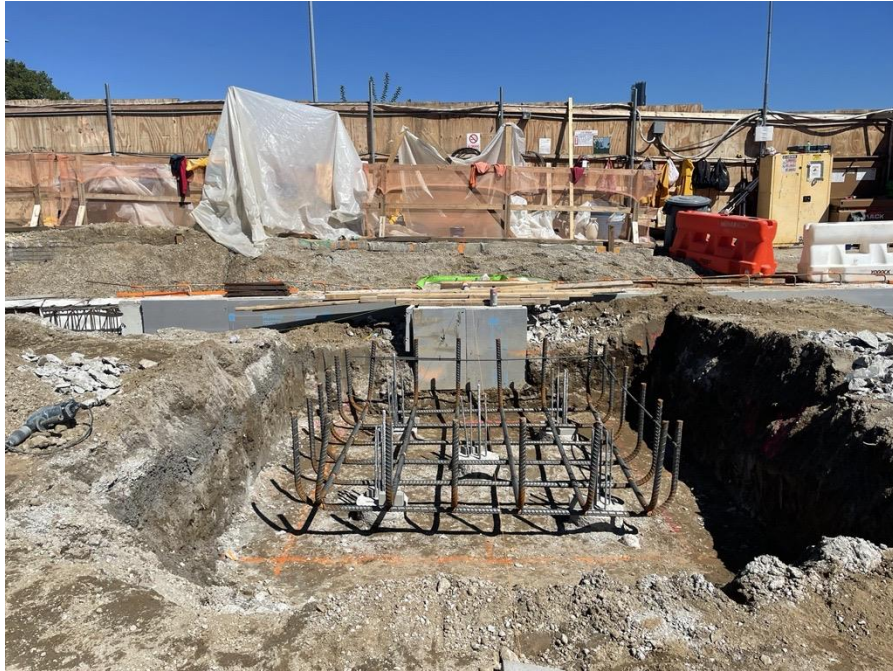
Photo 1: Bauer installing pile cap formwork in the northern part of the site (facing north).
