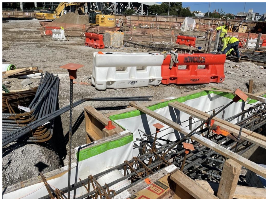
Photo 2: Bauer installing Preprufe 160R Plus within pile cap formwork prior to the pouring of concrete in the north-central part of the site (facing northwest).
