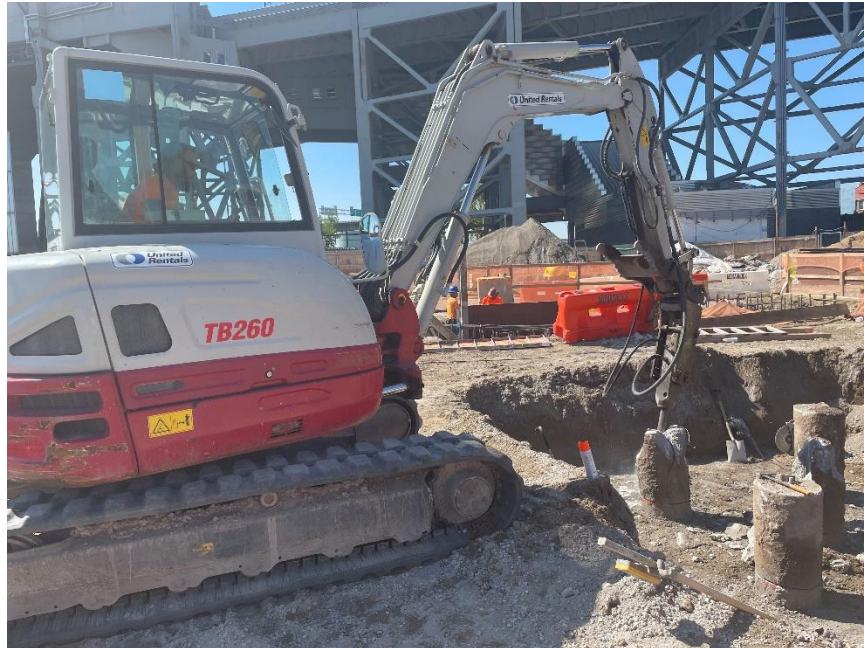
Photo 1: Bauer chopping existing concrete piles in the central part of the site (facing southeast)
