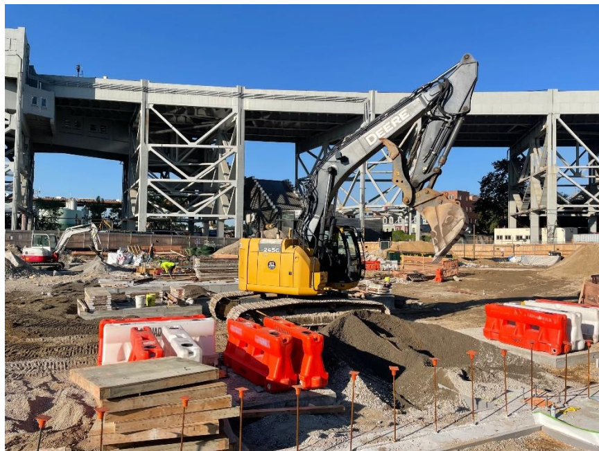
Photo 2: Bauer excavating in the north-central part of the site for formwork installation (facing southwest)
