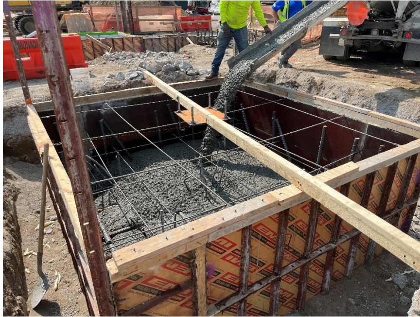
Photo 1: Bauer pouring concrete in the central part of the site (facing southeast).
