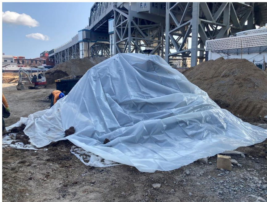
Photo 2: Bauer placing polyethylene sheeting on a stockpile in the western part of the site (facing southeast)
