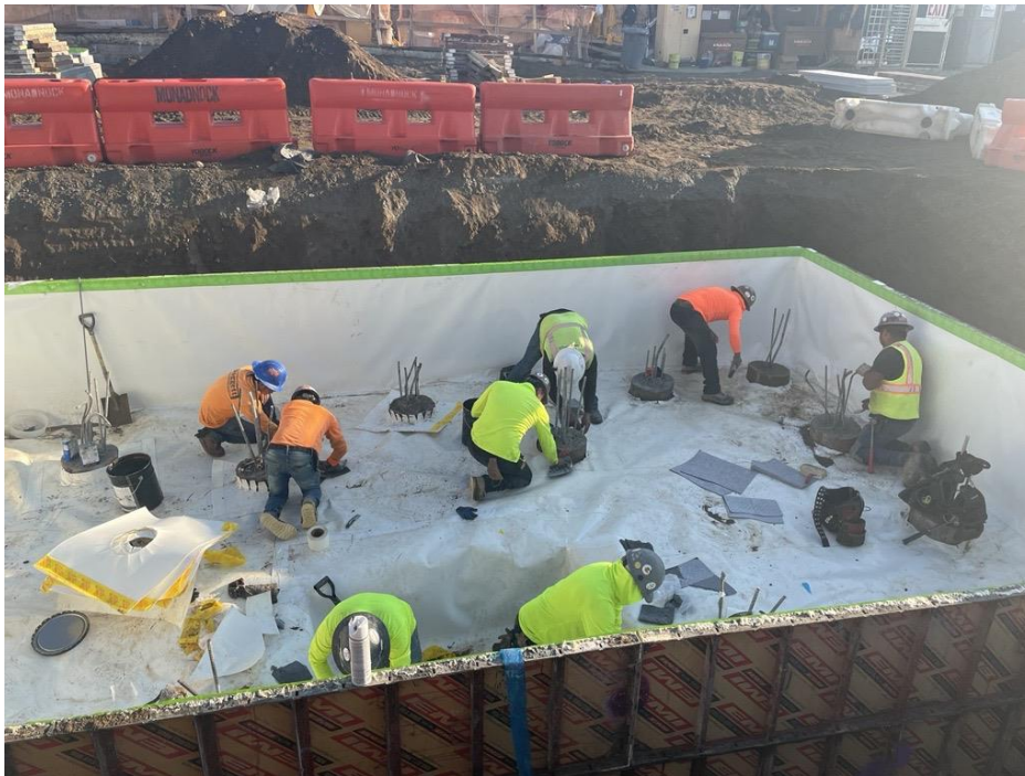
Photo 2: Bauer installing waterproofing/vapor barrier membrane (Preprufe 160R Plus on the vertical walls and Preprufe 300 on the horizontal surface at the base) within the elevator shaft in the central part of the site (facing north).
