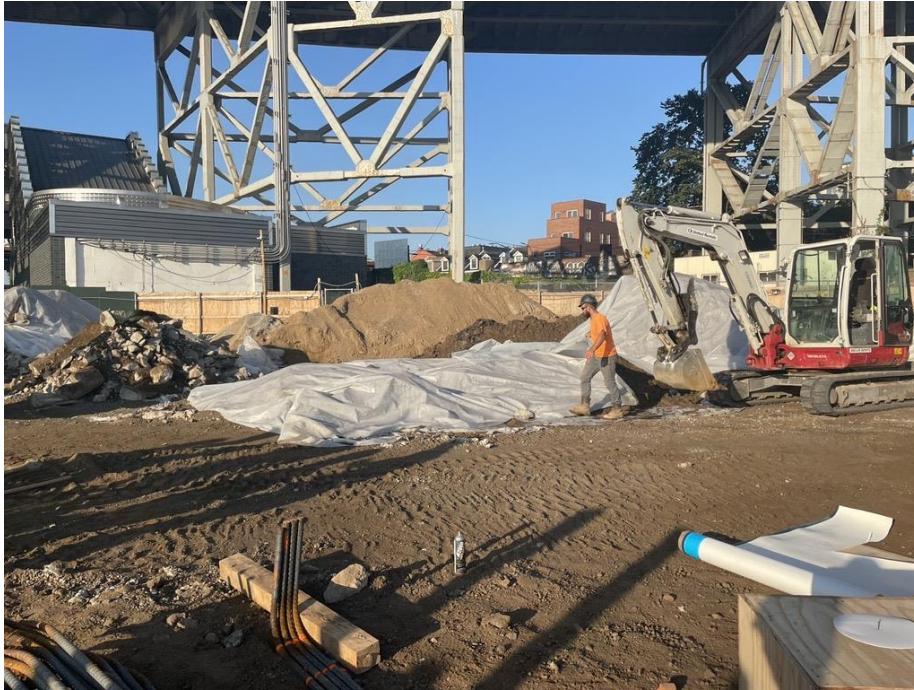
Photo 1: Bauer covering a stockpile with polyethylene sheeting in the southwestern part of the site (facing southwest)
