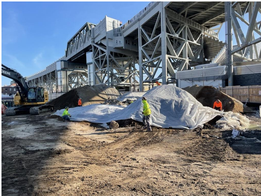
Photo 2: Bauer covering a stockpile with polyethylene sheeting in the southwestern part of the site (facing southeast)
