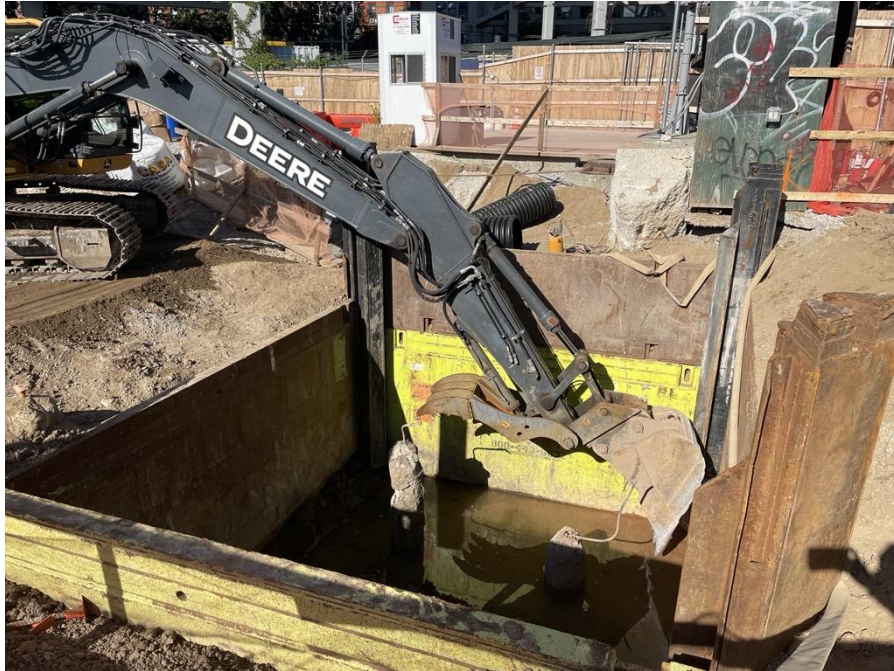
Photo 1: Bauer excavating within the shoring box in the northwestern part of the site (facing west).
