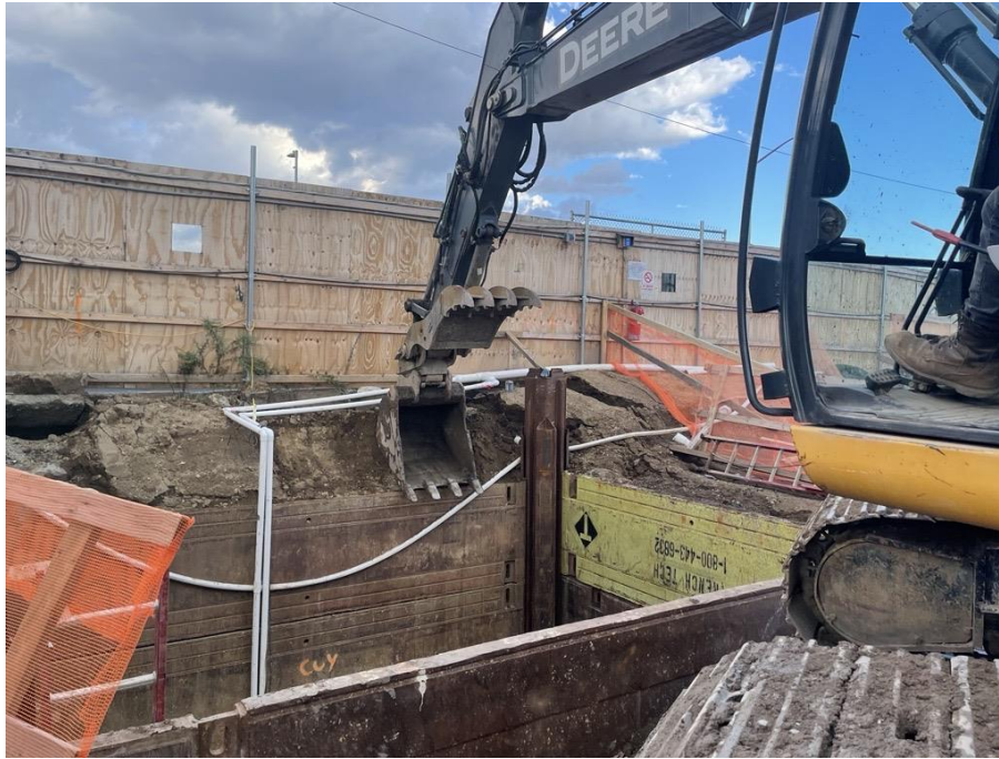
Photo 1: Bauer excavating in the shoring box (facing northeast).
