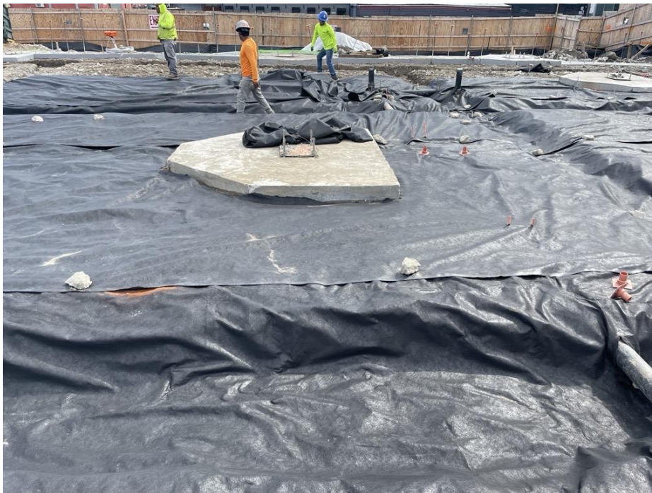
Photo 2: Bauer installing filter fabric in the southeastern part of the site (facing east).
