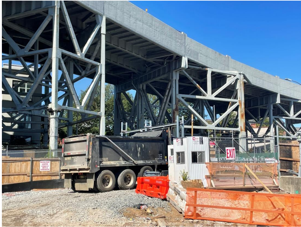
Photo 1: Truck with tight fitting cover exporting soil from the site (facing northwest).
