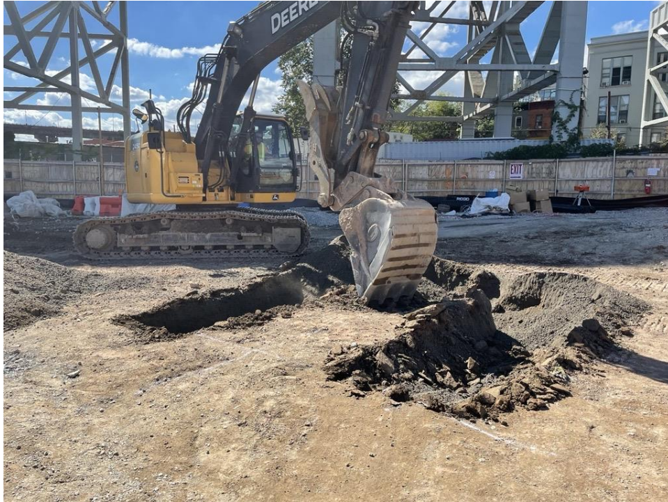
Photo 2: Bauer excavating for pile caps in the western part of the site (facing southwest).
