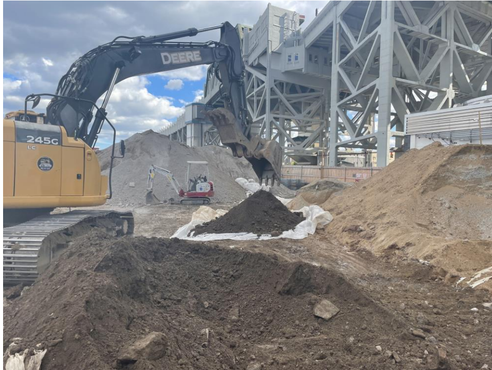
Photo 2: Bauer relocating a stockpile in the southern part of the site (facing southeast).
