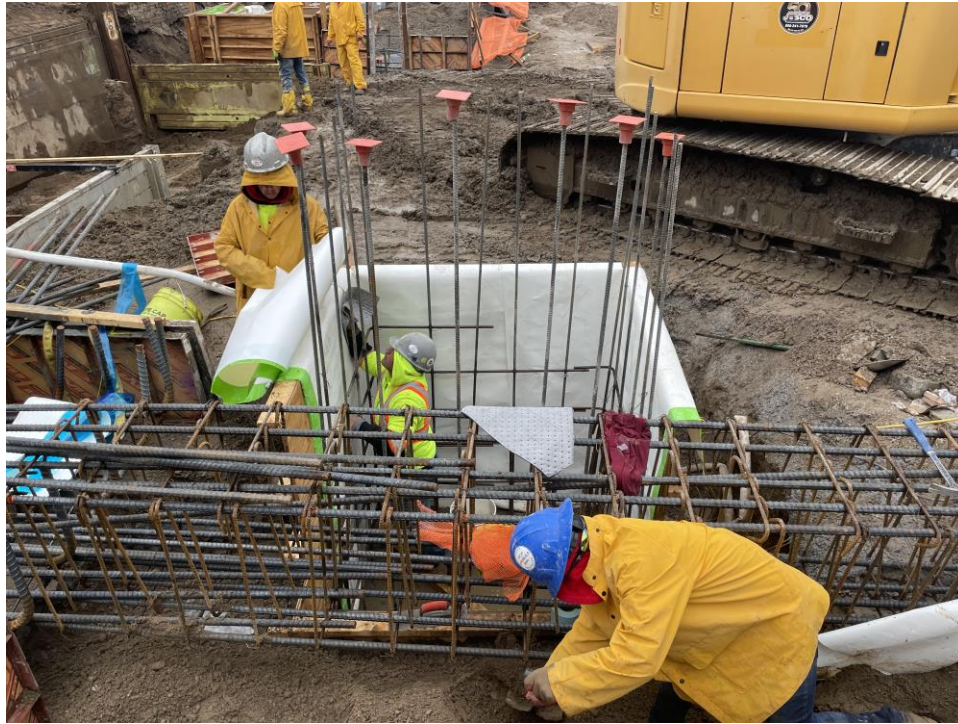
Photo 1: Bauer installing waterproofing/vapor barrier membrane (Preprufe 160R Plus) on the vertical walls within the formwork in the western part of the site (facing east).
