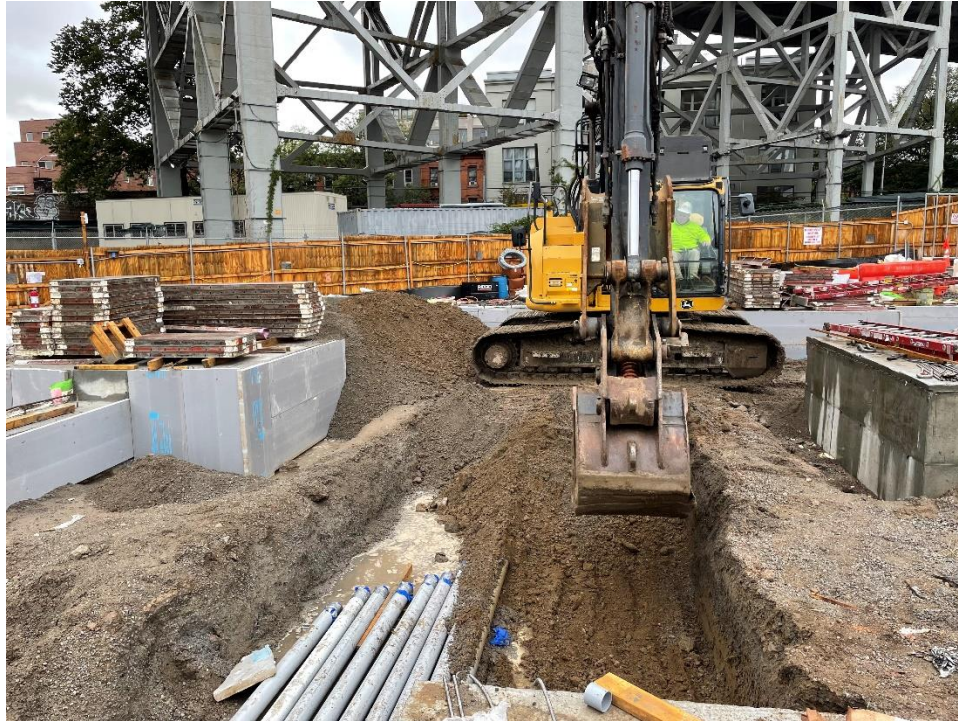
Photo 2: Bauer excavating in preparation for electrical piping installation in the western part of the site (facing southwest).
