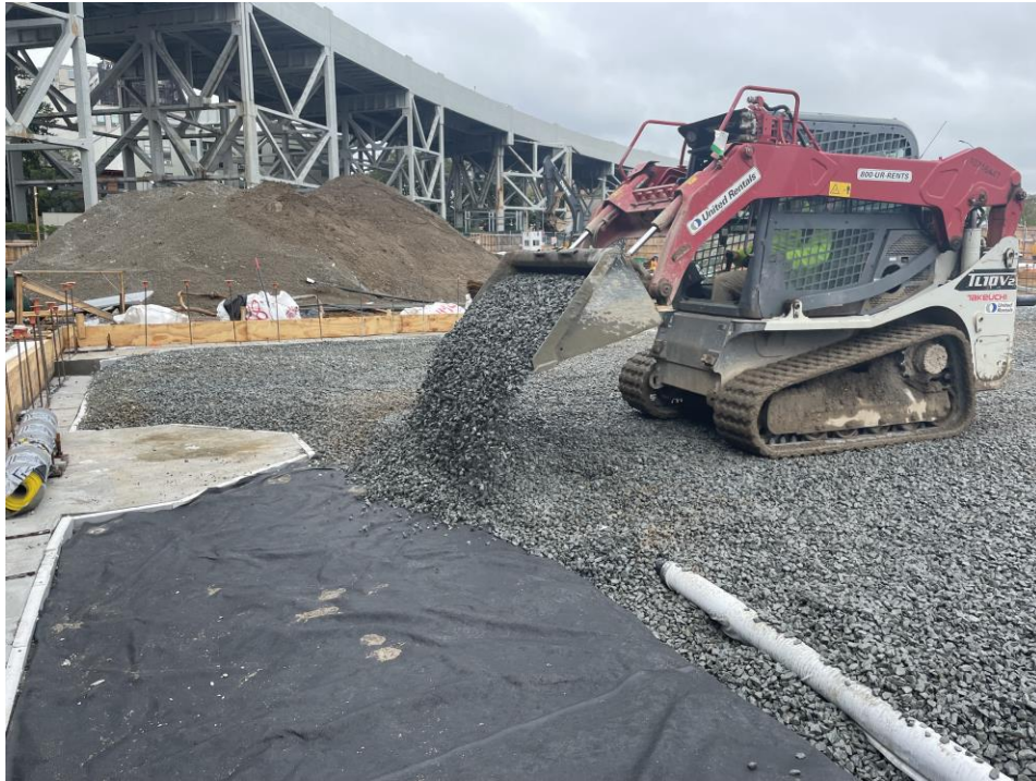
Photo 1: Bauer backfilling with previously imported and stockpiled ASTM #5 stone for the installation of the sub-slab depressurization system in the southeastern part of the site (facing west).
