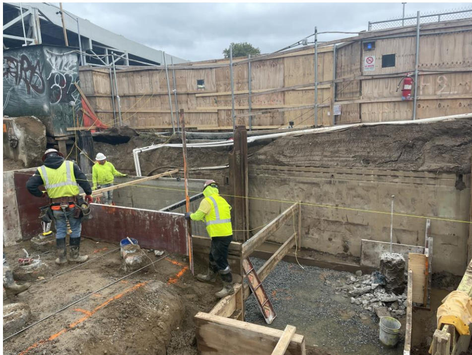
Photo 2: Bauer installing formwork in the western part of the site (facing north).
