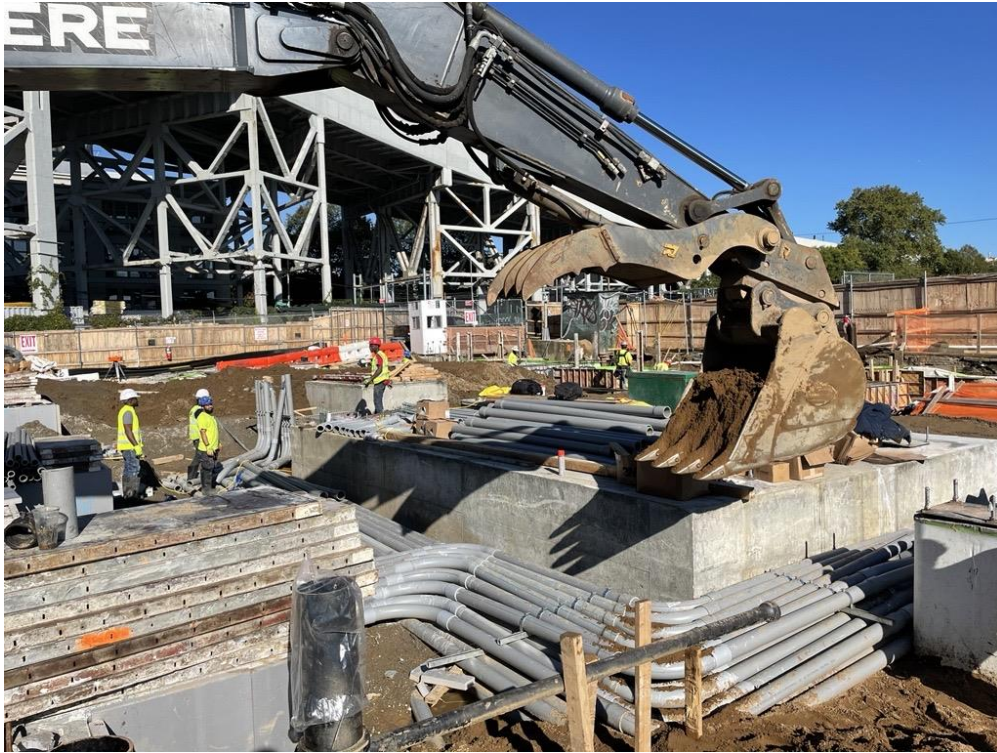
Photo 1: Bauer backfilling with previously imported and stockpiled clean fill over the electrical conduits in the central part of the site (facing northwest).
