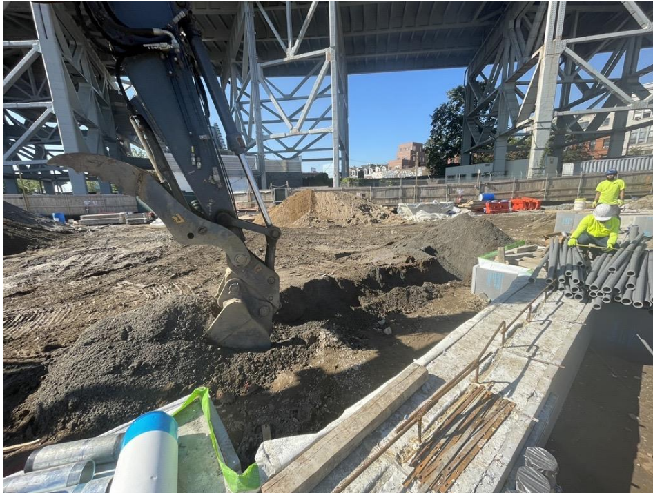
Photo 1: Bauer excavating a trench in the central part of the site for plastic electrical conduit installation (facing south).
