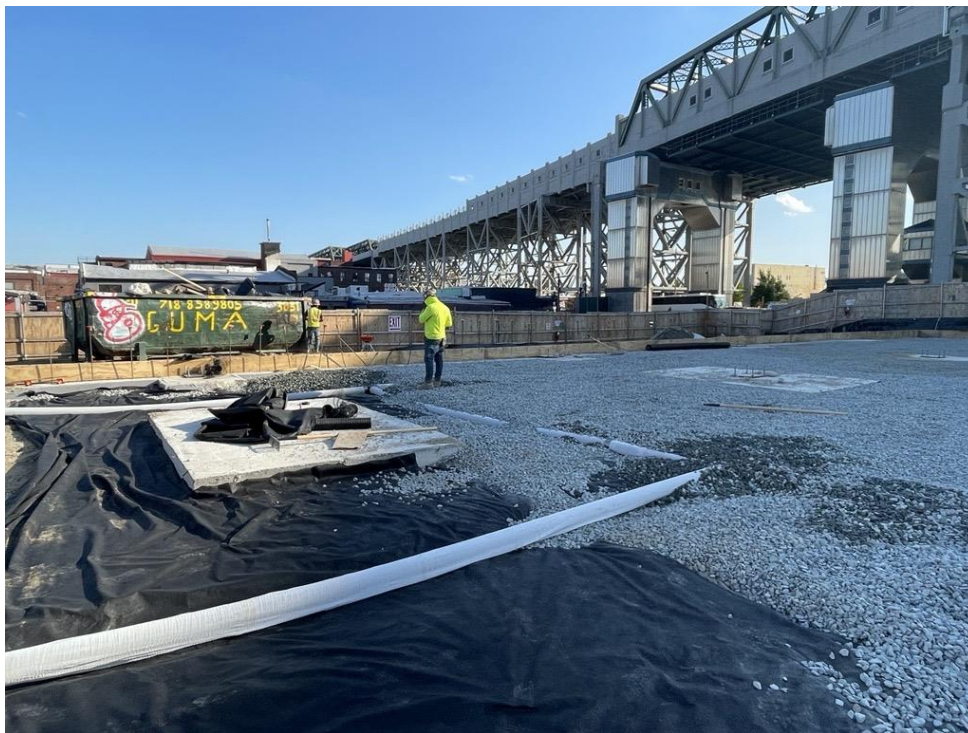
Photo 2: Bauer installing the SMD system in the southeastern part of the site (facing east).
