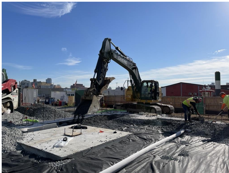
Photo 2: Bauer backfilling with previously imported and stockpiled ASTM #5 stone for the installation of the SMD system in the northeastern part of the site (facing northeast).
