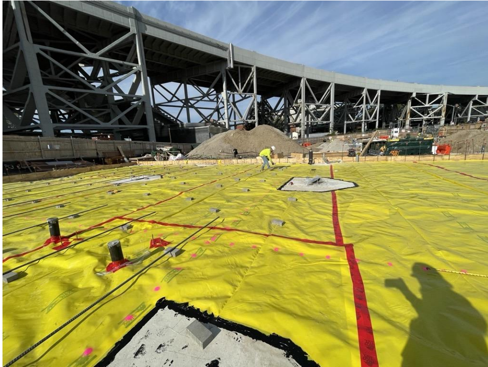
Photo 1: Bauer installing Stego® Wrap 20-mil Vapor Barrier as part of the SMD system in the southeastern part of the site (facing southwest).
