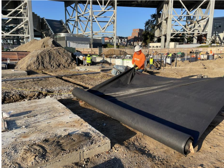
Photo 1: Bauer installing filter fabric as part of the SMD system in the northeastern part of the site (facing southwest).
