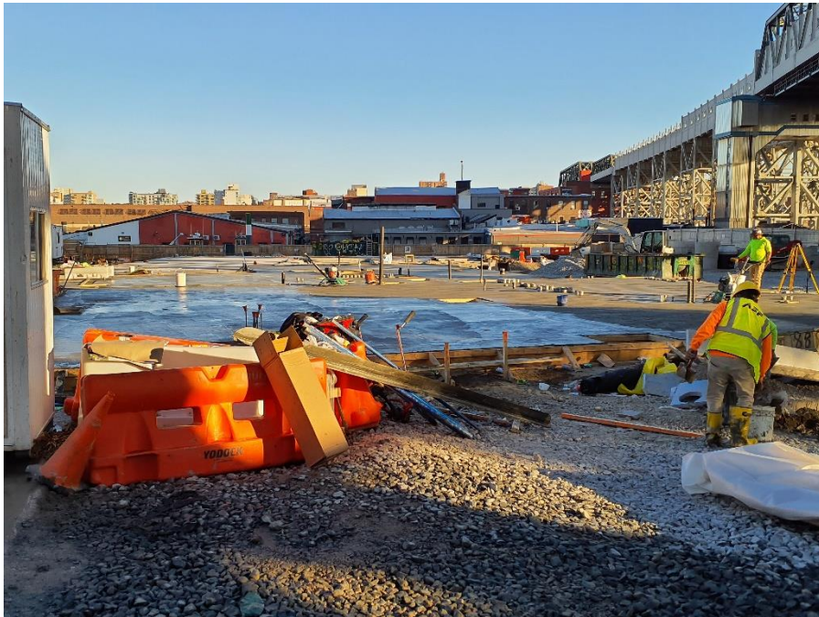
Photo 2: General view of the poured foundation slab (facing east).
