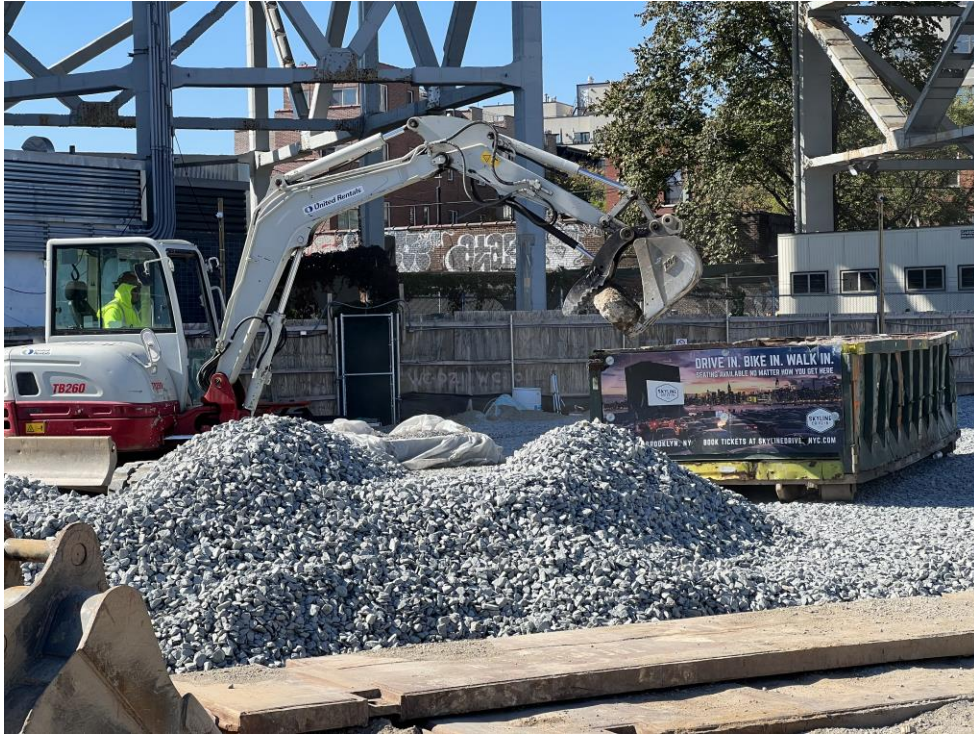
Photo 1: Bauer stockpiling C&D in a rolloff container (facing south).
